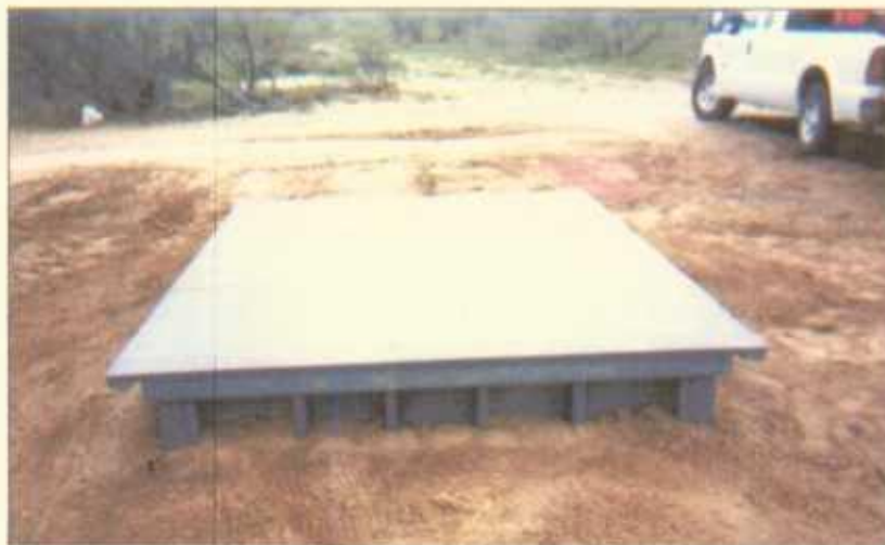
Completed Junction Box
