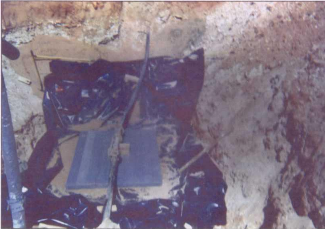
Construction of New Junction Box With Poly Liner
