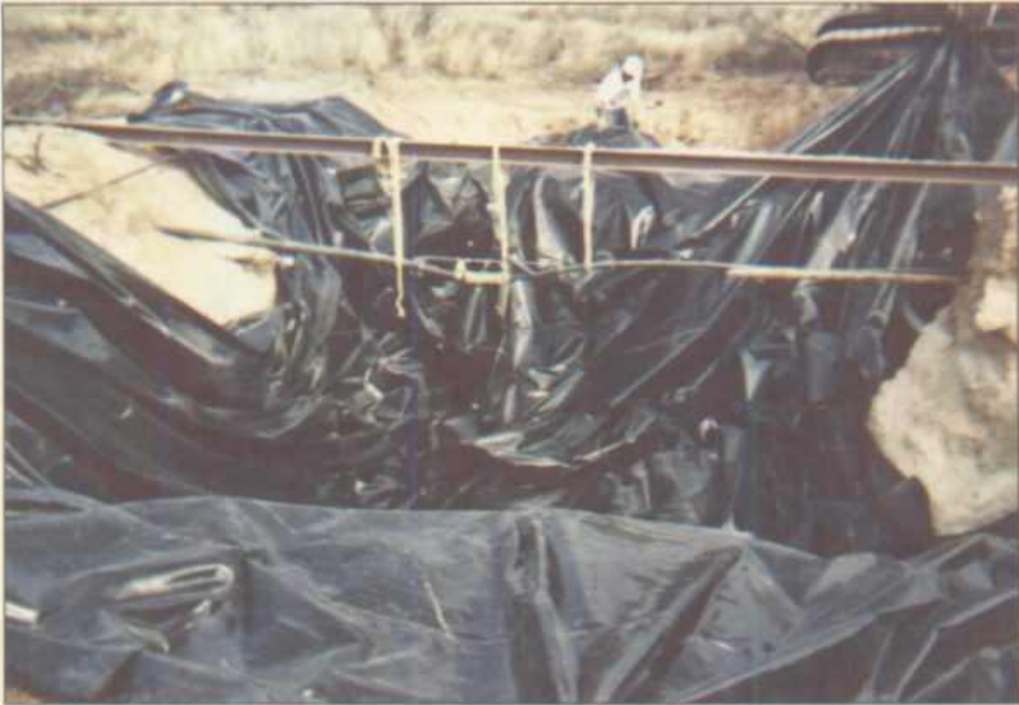
Installation of 20 mil Poly Liner
