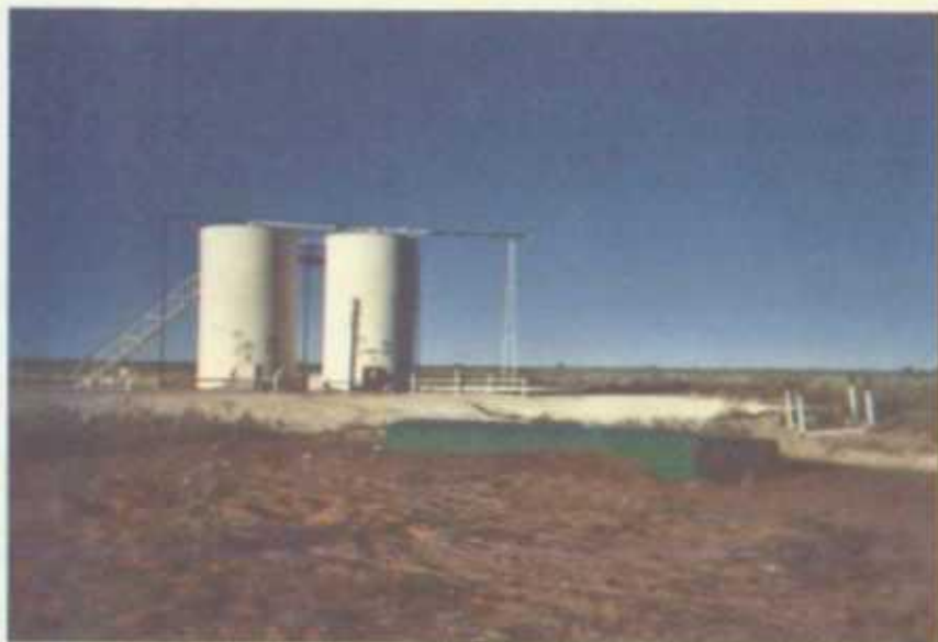
Undisturbed Junction Box
