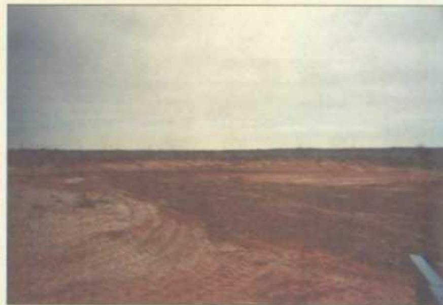
Backfilled excavation looking SE from new box
