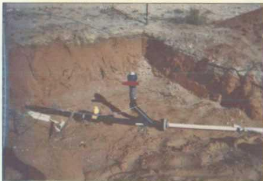
New plumbing at new box site 70 ft NW of old one
