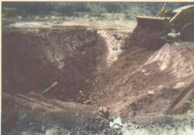
Impact Excavation with Clay Barrier
