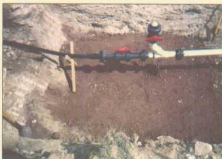
New Plumbing for New Box (with clay barrier)
