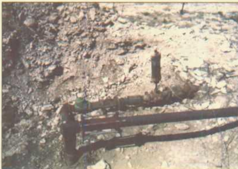
NORM Removal With Old Plumbing
