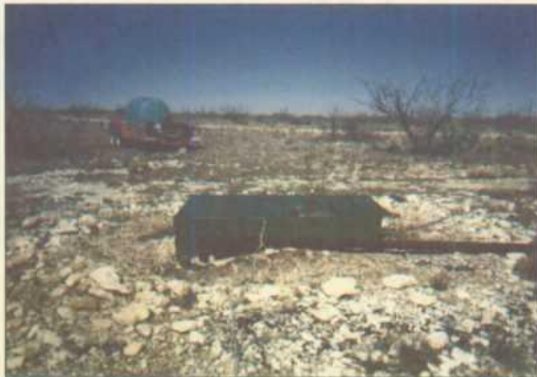
Old Junction Box
