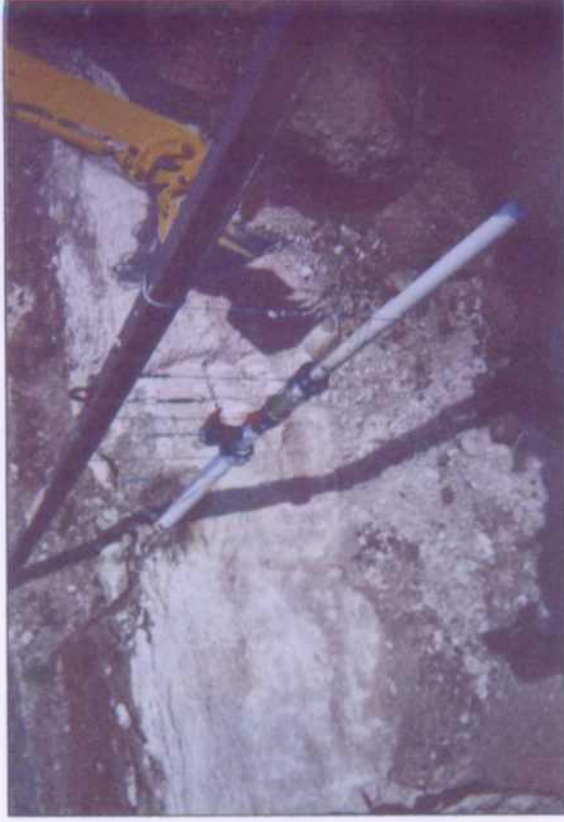
25 ft x 20 ft x 15 ft deep Excavation (June 2003)
