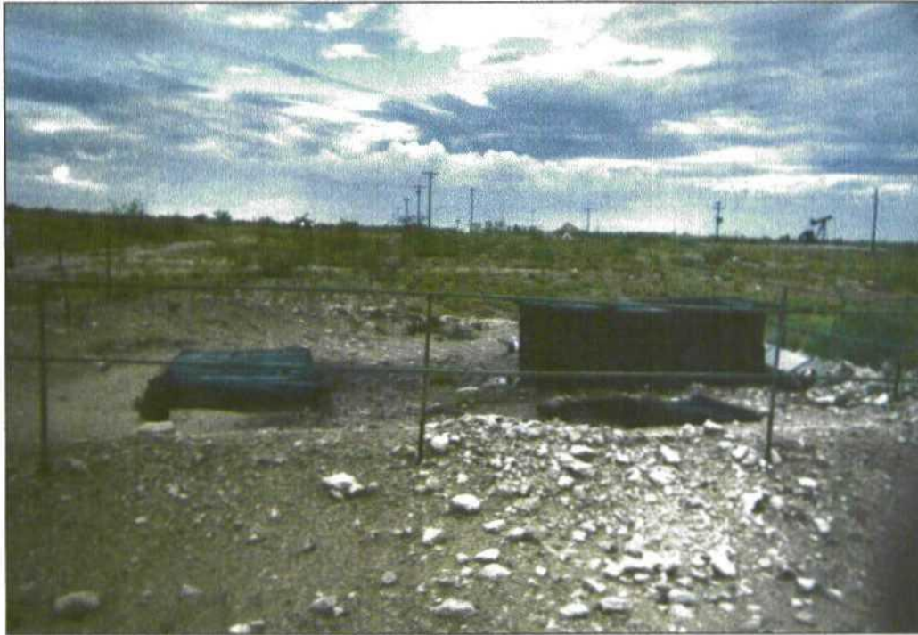
Undisturbed junction box 4/8/2003
