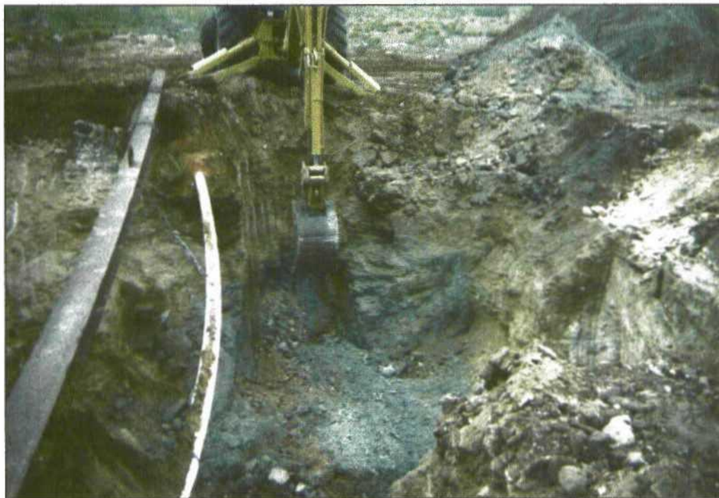
Excavation at old junction Nov. 2003
