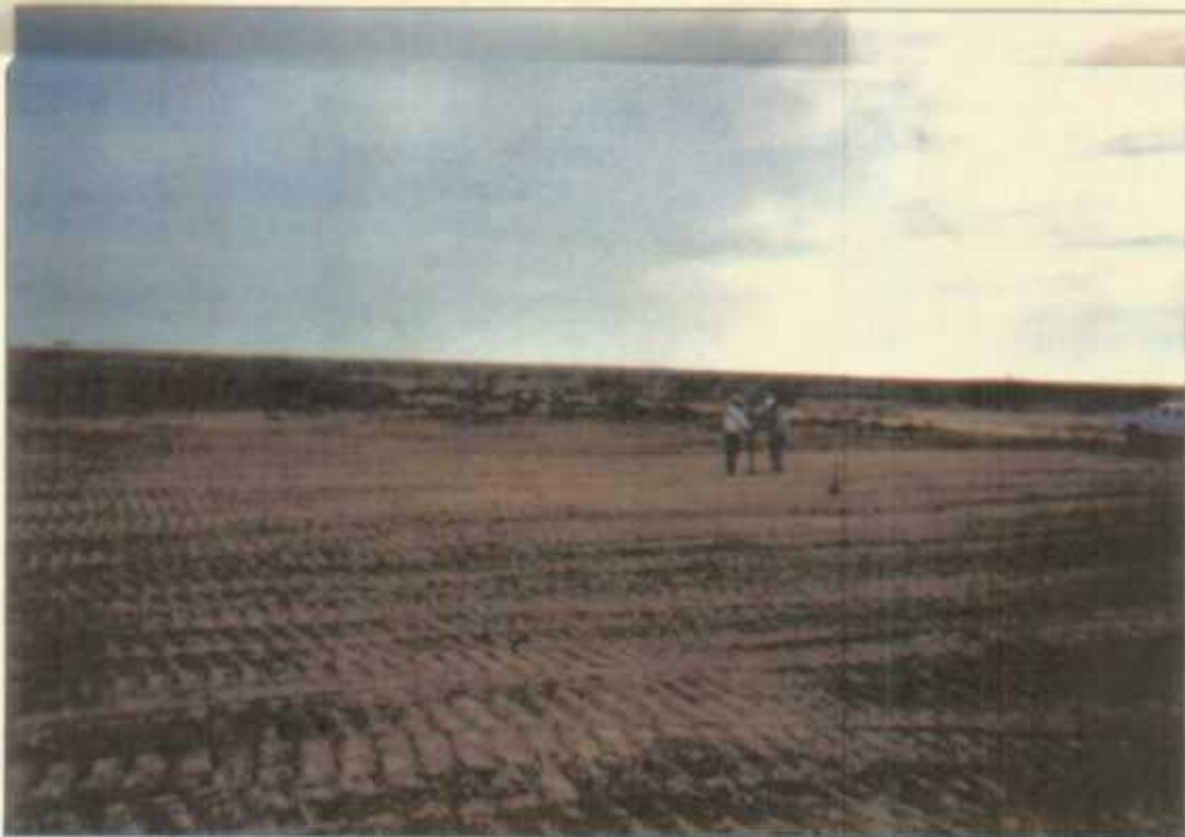
Backfilled (looking north)
