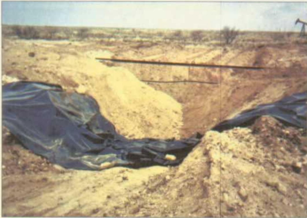
Backfilling Poly Liner
