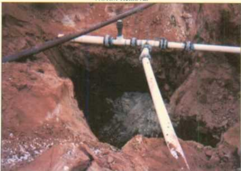
Remediation (with new plumbing)
