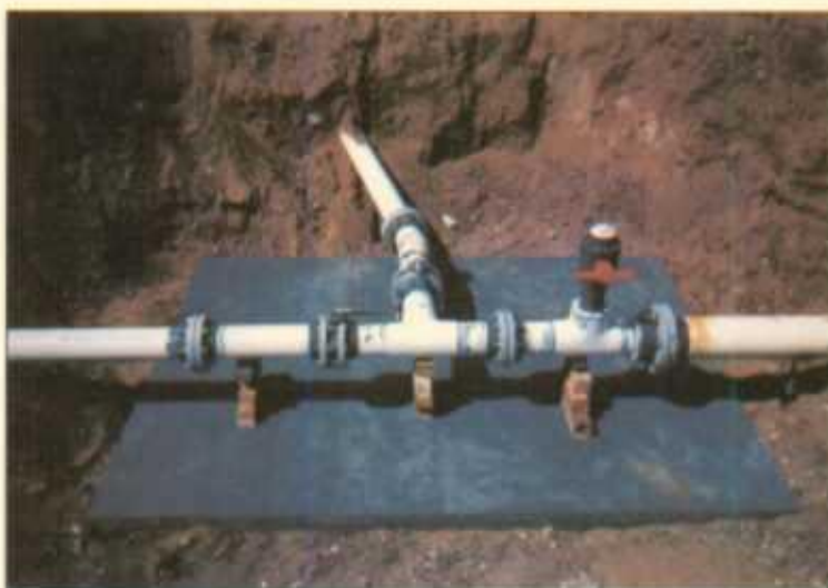
New Box Construction
