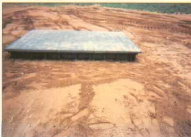
Completed Junction Box
