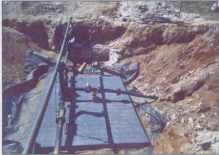
New Box Construction with Poly Liner
