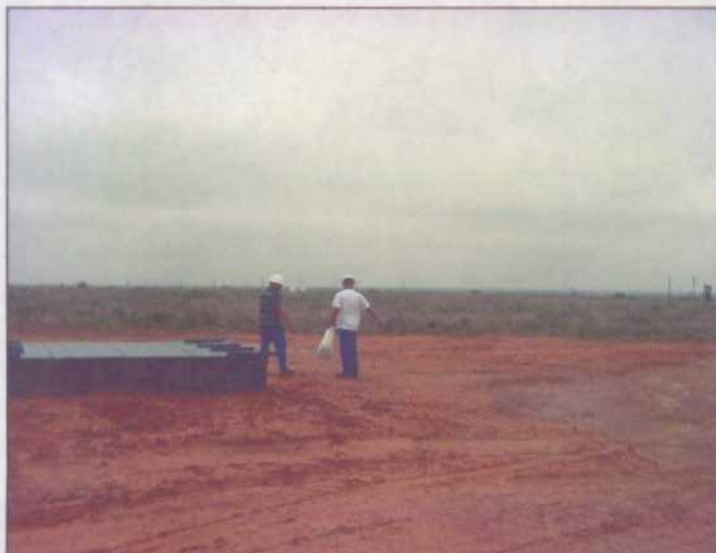
Seeding New Topsoil
