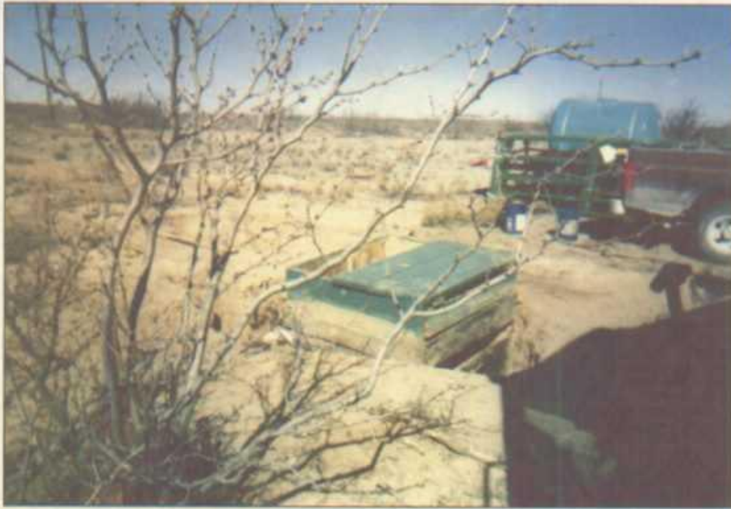
Old jct. box (NORM removal)
