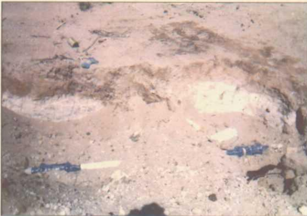
New plumbing after NORM removal
