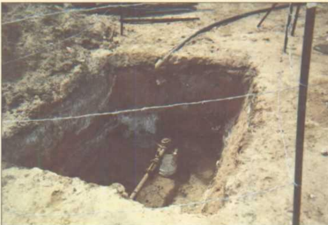
After NORM Removal; Before Remediation
