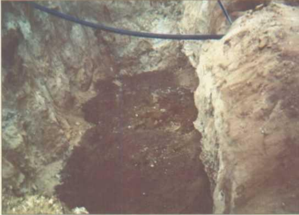
Excavation with Clay Liner at Bottom
