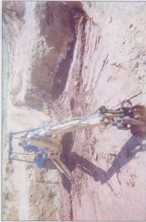
installing and compacting clay barrier at 6 ft BGS 5/11/2004
