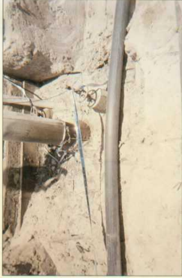
former junction site; box removed; poly pipeline straight through 6/6/2004
