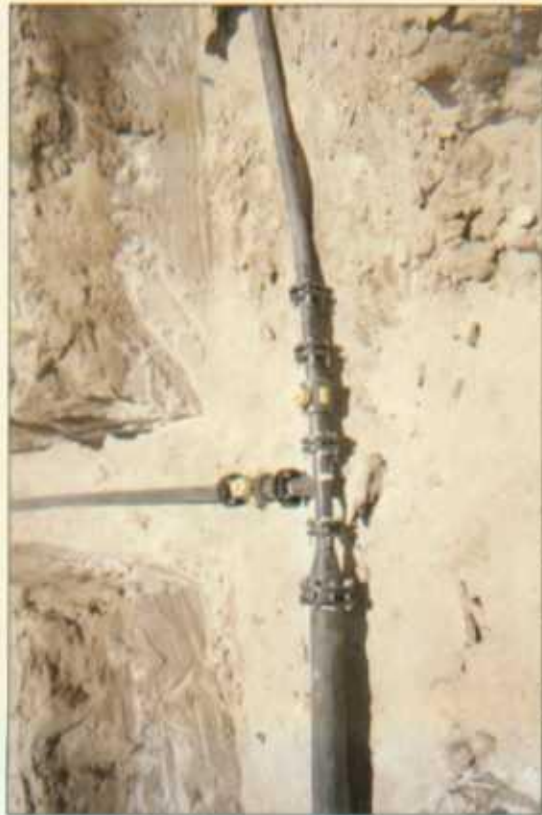
new poly junction 15 ft east of former junction 6/6/2004
