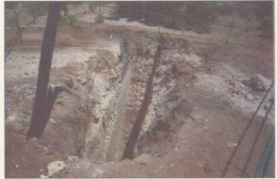
Vertical Delineation Excavation At Old Jct. Site—7/22/2003
