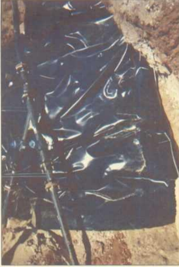
Installing 20 mil Poly Liner
