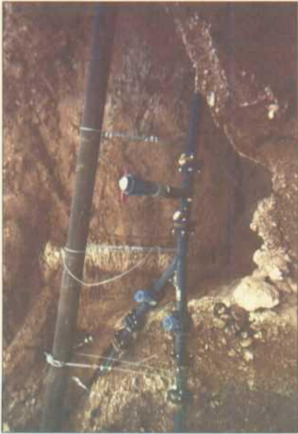
Backhoe Excavation May 2003
