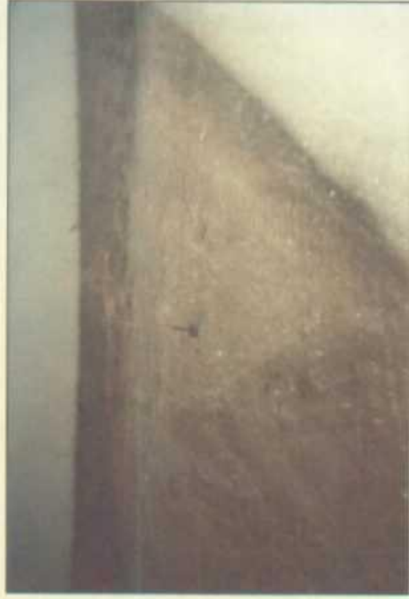
Shovel marking plate to identify clay barrier below
