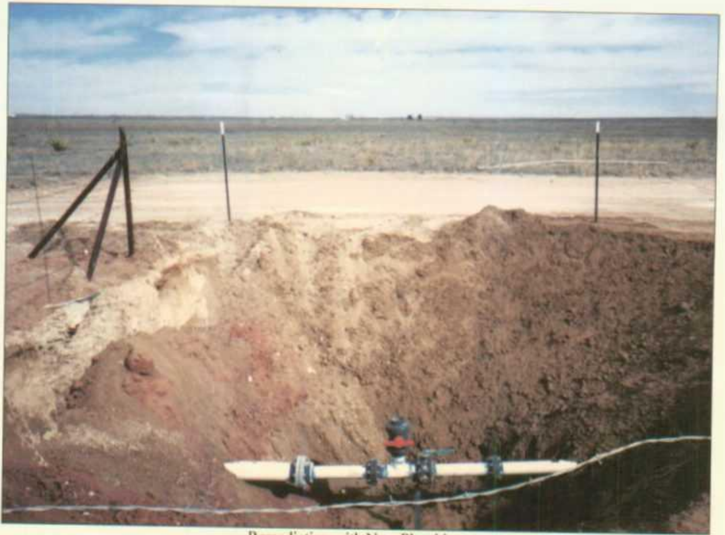
Remediation with New Plumbing
