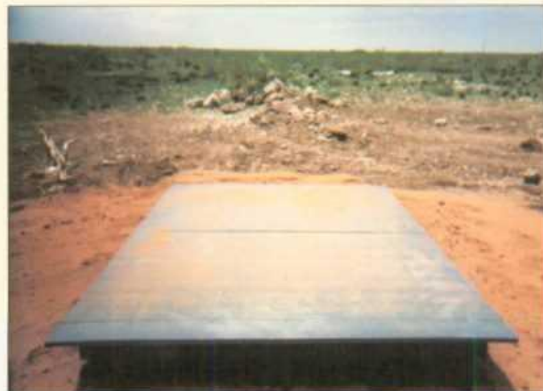
Completed Junction Box
