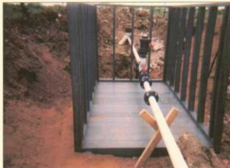
New Box Construction
