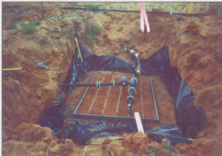
Construction of Box Floor With Poly Liner
