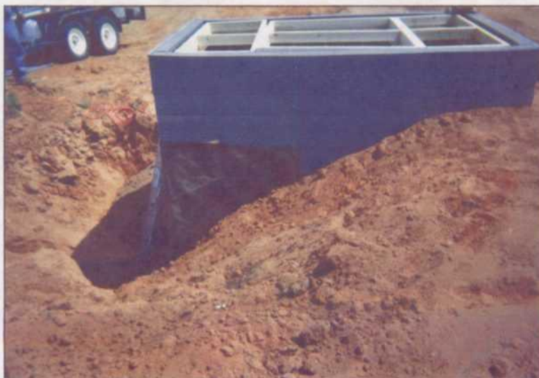
New Box Construction
