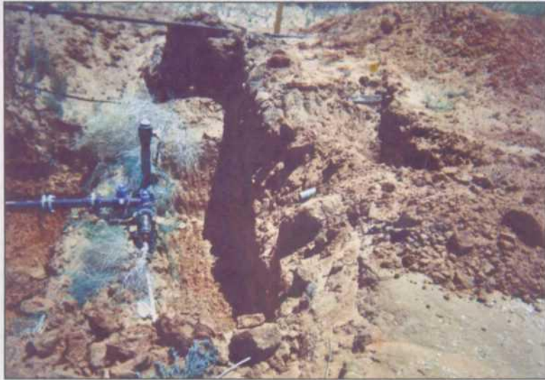
After NORM Decontamination & New Plumbing
