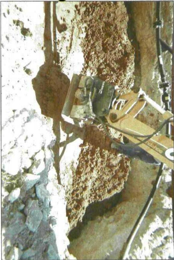
compacting clay barrier at 6 ft BGS
