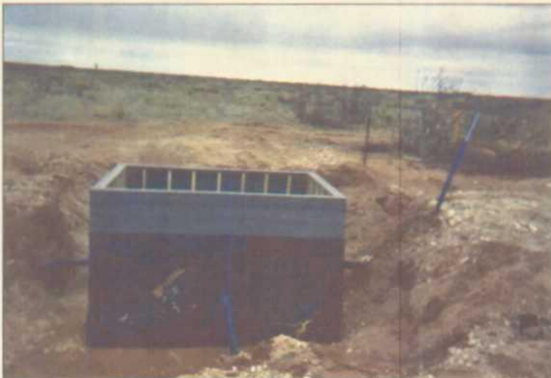
Construction of New Jet. Box
