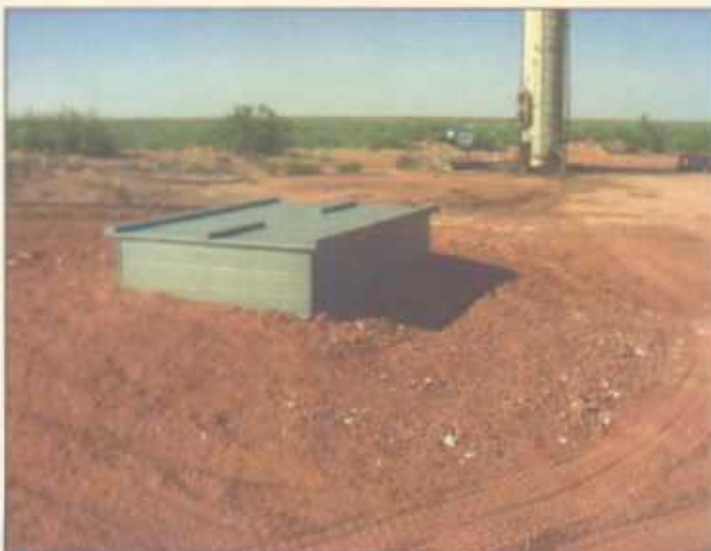
Backfilled With New Junction Box
