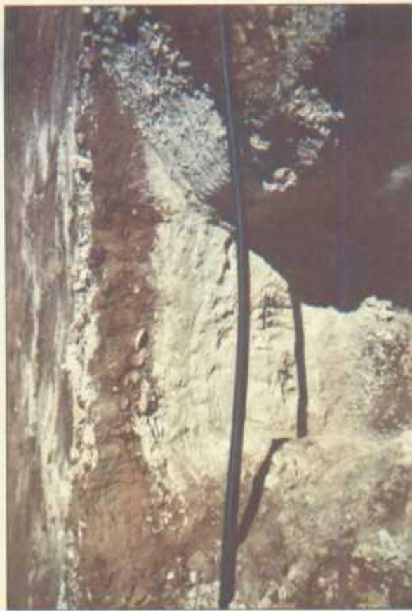
10 x 10 x 12-ft-deep Excavation July 2003
