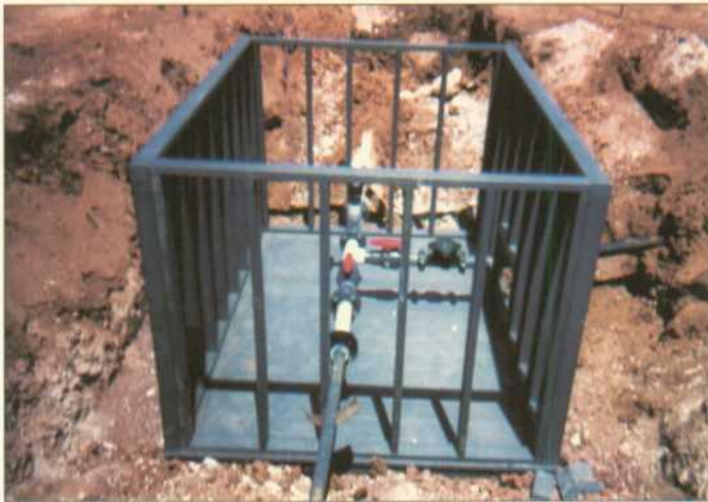
New Junction Box Construction
