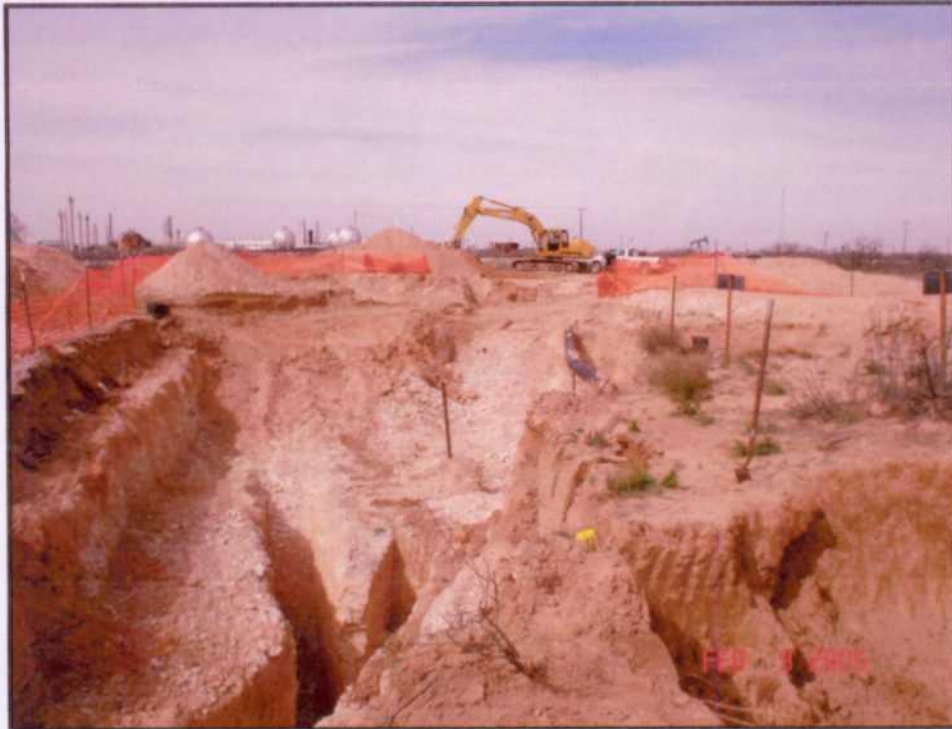
Northwest view of excavation after removing pipeline.
