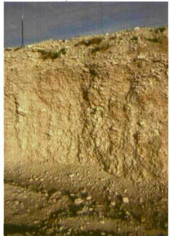
*Figure 3 - Wall of the excavation shows upper 10-13 feet of the vadose zone.*
