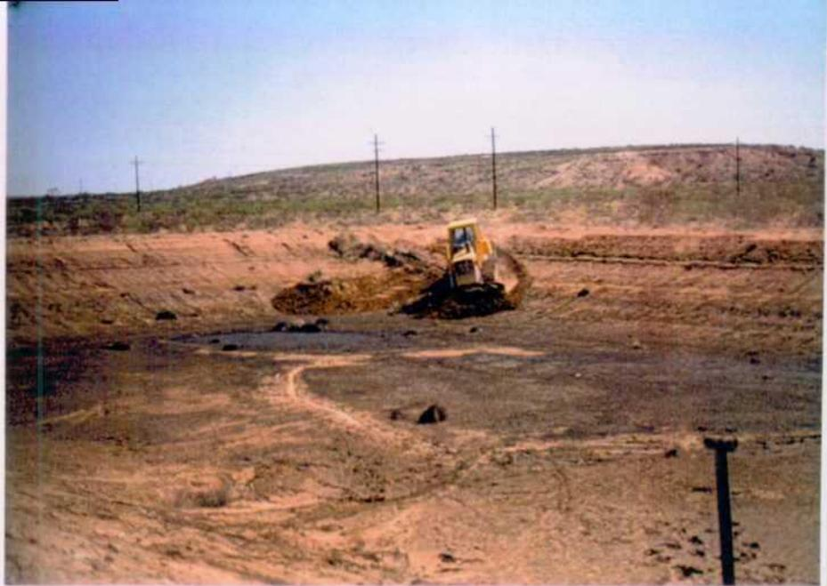
5. Excavation of heaviest section of sludge to 4 feet deep
