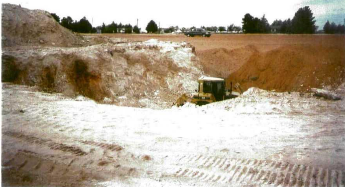
1. Pipeline Excavation – Hydrocarbon Staining Near Center of South Wall Beneath Pipeline
