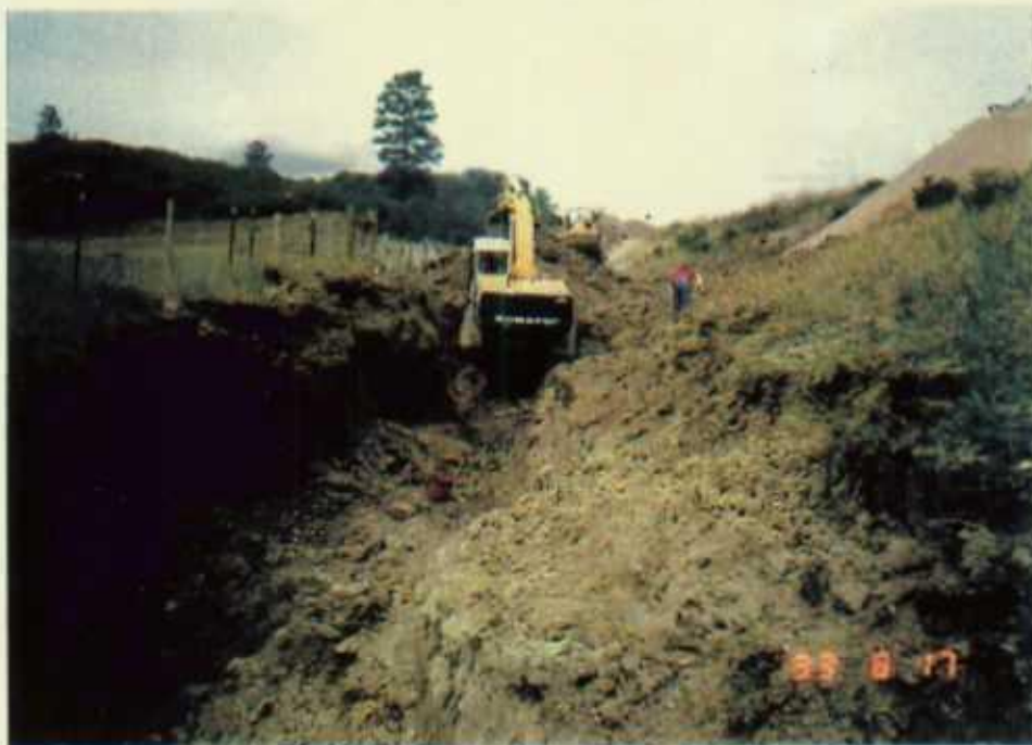
EXCAVATION - LOOKING NORTH
