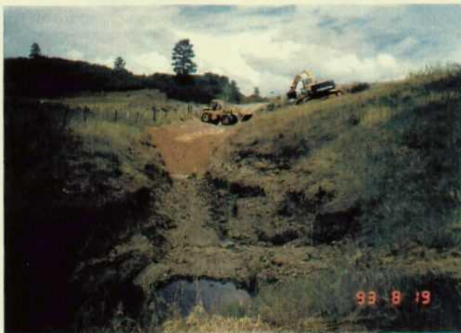
BACKFILLING IN PROGRESS - LOOKING NORTH
