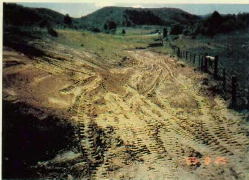
COMPLETED RECLAMATION - LOOKING NORTH
