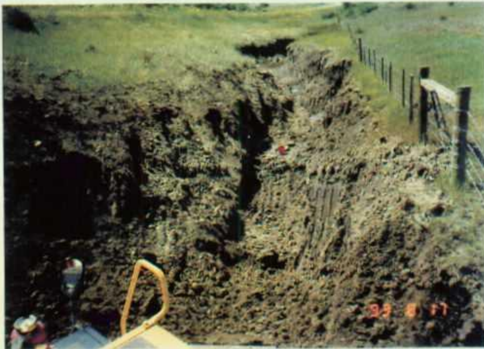
EXCAVATION - LOOKING SOUTH
