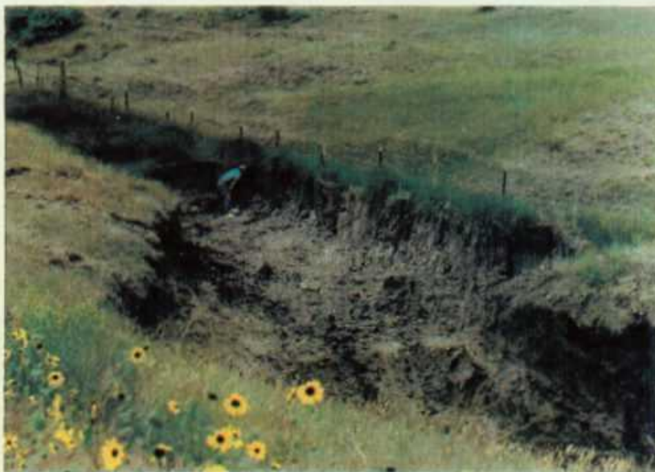
SOUTH END OF EXCAVATION
