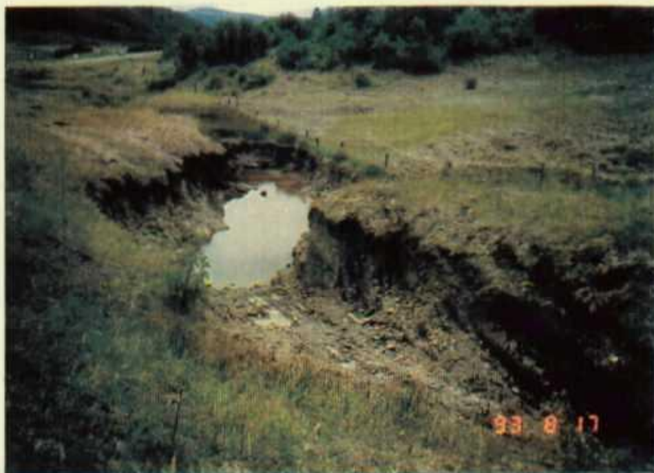
SOUTH END OF EXCAVATION AFTER INFILTRATION OF METEORIC WATER
