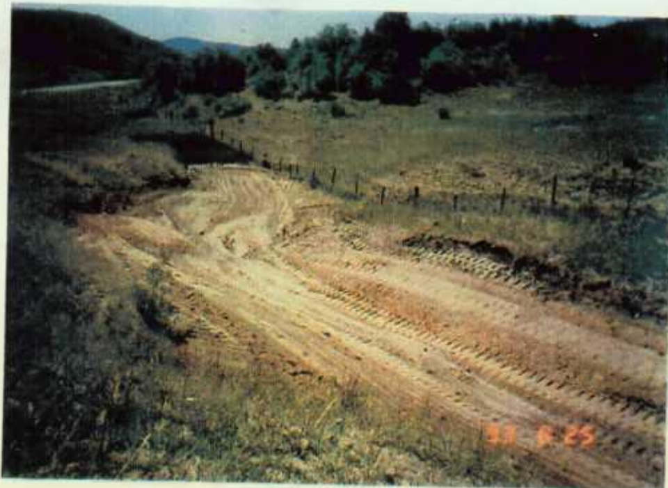
SOUTH END OF COMPLETED RECLAMATION
