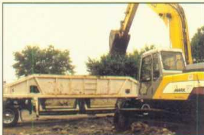
Excavated material loaded onto truck for transport to landfarm
