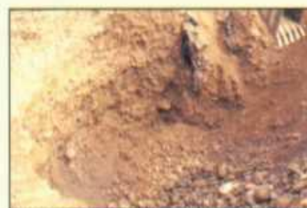
Overexcavation of hydrocarbon stained soil
