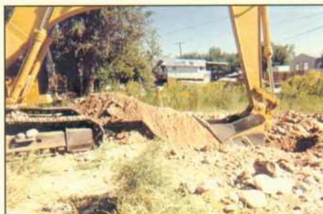
Looking NE Initial excavation showing dark brown sand and cobbles
