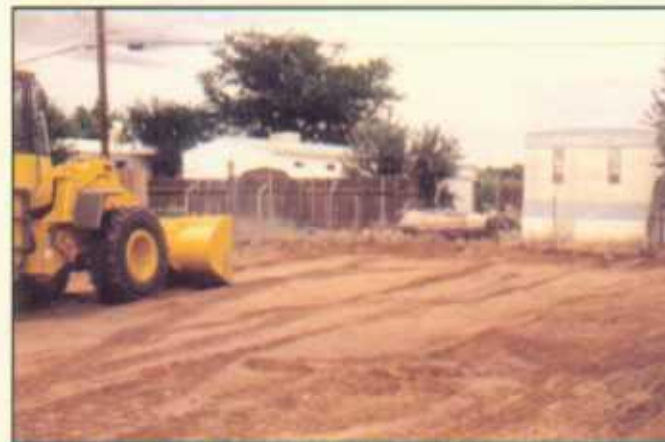
Looking East, cleanfill compacted and graded to ground surface
