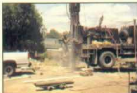
Installation of monitor well MW-01
