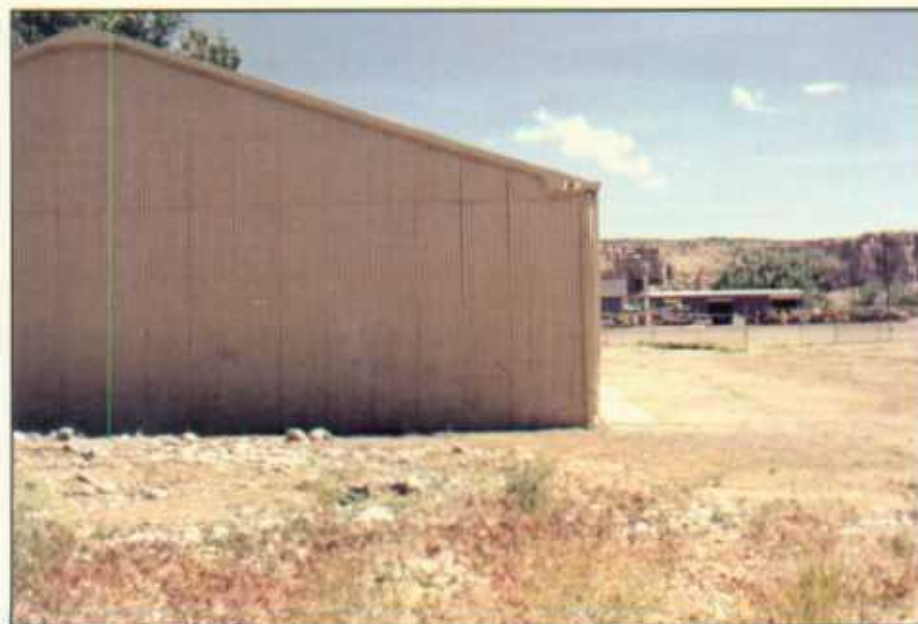
North of building prior to excavation
