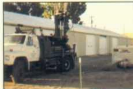
Installation of monitor well MW-04
