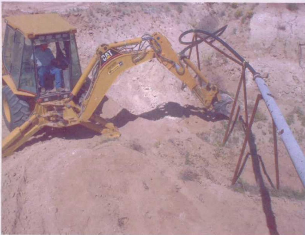
Floor excavation from East wall
