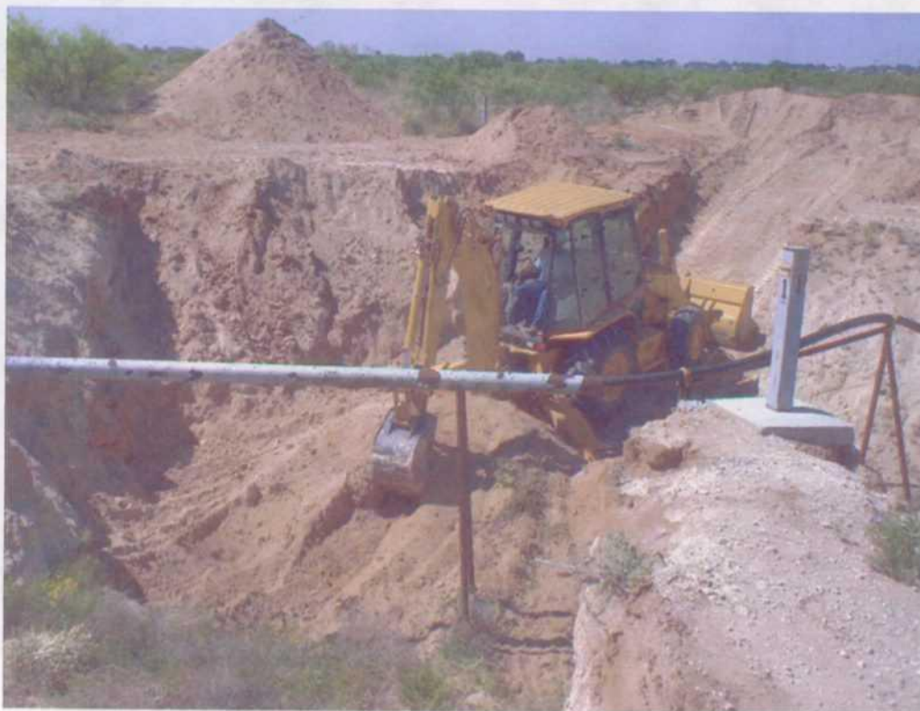
Looking South from Northeast wall toward South wall and ramp, monitor well MW-1 in foreground
