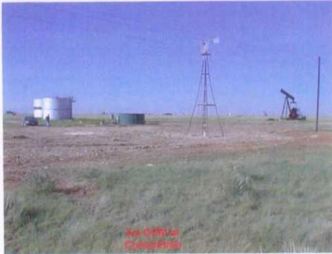
An example of a site in which the contamination from a pit impacted a shallow aquifer. We were able to drill a recovery well in the center of the impoundment, install a windmill complete with down-hole oil / water separator and pump the free product directly into a temporary storage tank at a fraction of the cost of traditional pump and treat methods.
