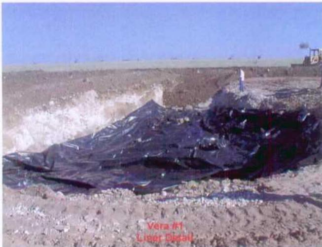
Many impoundments may be closed by means of encapsulating the contaminated soils within a high-density polyethylene liner. Typically, a water monitoring well is installed immediately down gradient from the site to insure liner integrity.
