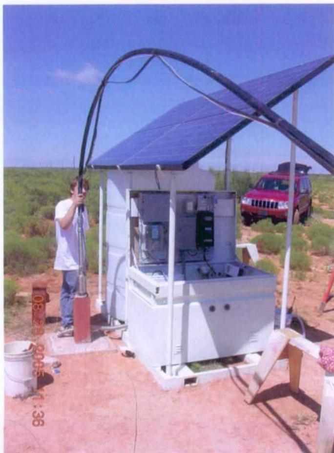
**Example of our remote R.O. Treatment system. Powered exclusively by sun and wind, the unit pumps water from the aquifer into a storage tank. The fluid is treated through reverse osmosis producing up to 95% clean, potable water and 5% super-saturated brine.**
