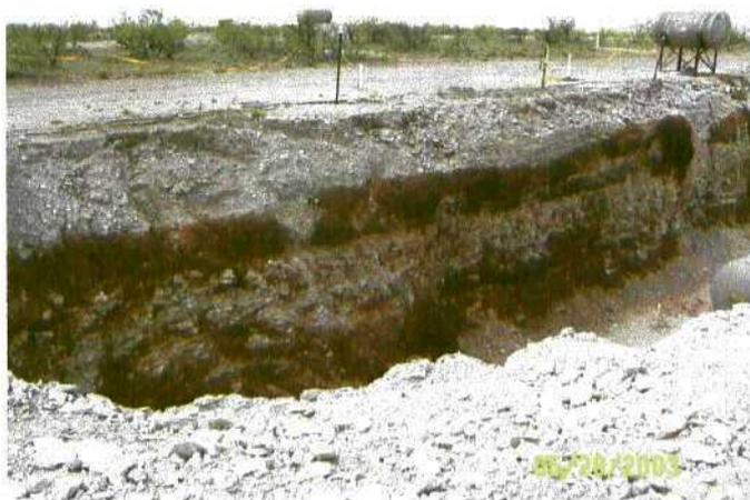
A different view of the site showing the areas of migration of the oil from the leaking pipeline. The pipeline in question was installed only 18 months prior to the leak.
