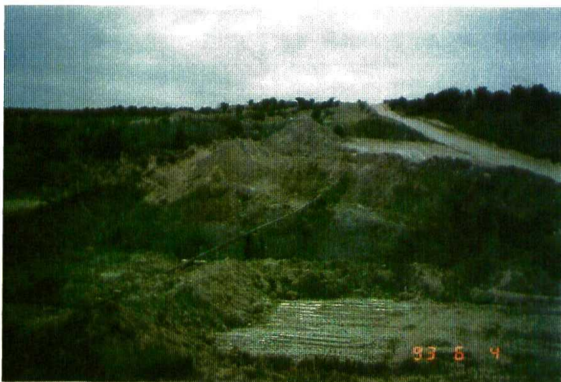
FINAL EXCAVATION-LOOKING EAST
