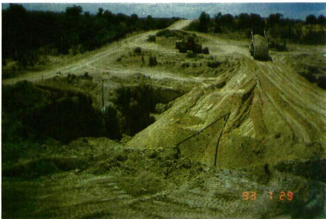
BACKFILLING OF EXCAVATION LOOKING WEST
