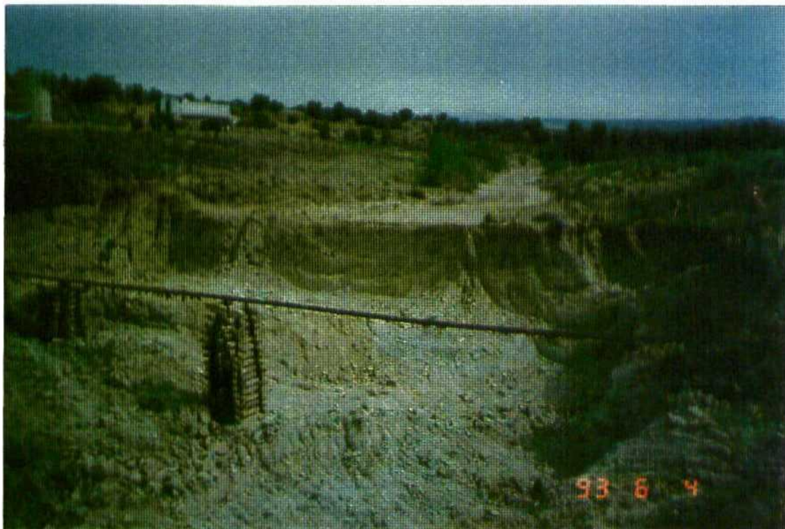
FINAL EXCAVATION-LOOKING NORTH
