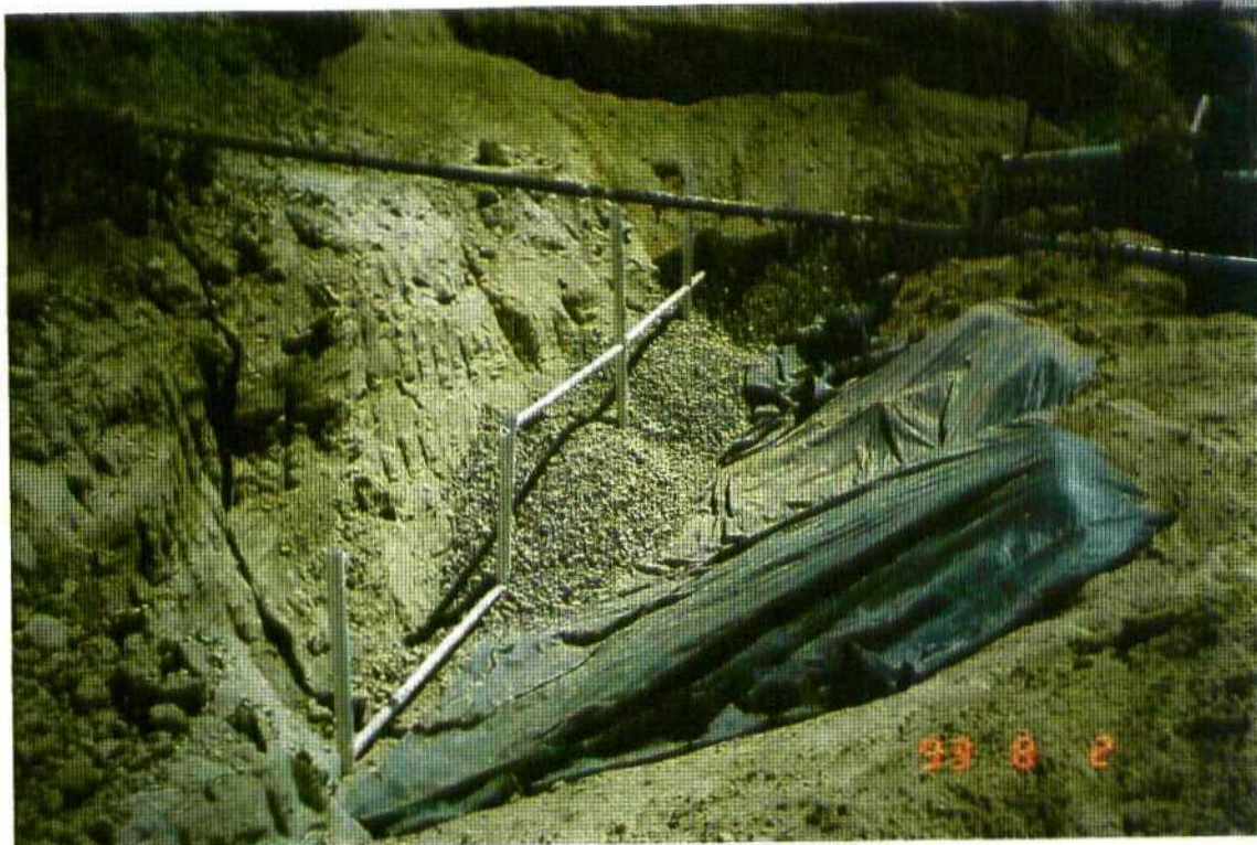
SOIL VAPOR EXTRACTION (SVE) SYSTEM INSTALLATION
