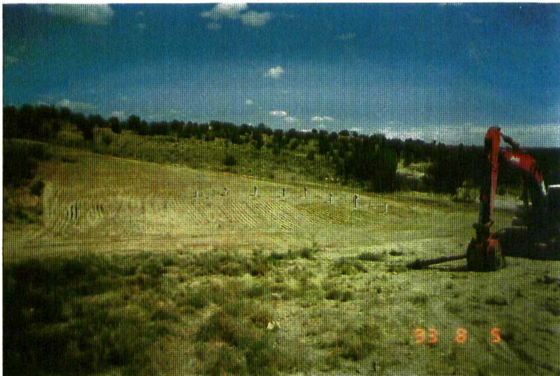
FINAL SITE RECLAMATION-LOOKING SOUTHEAST
