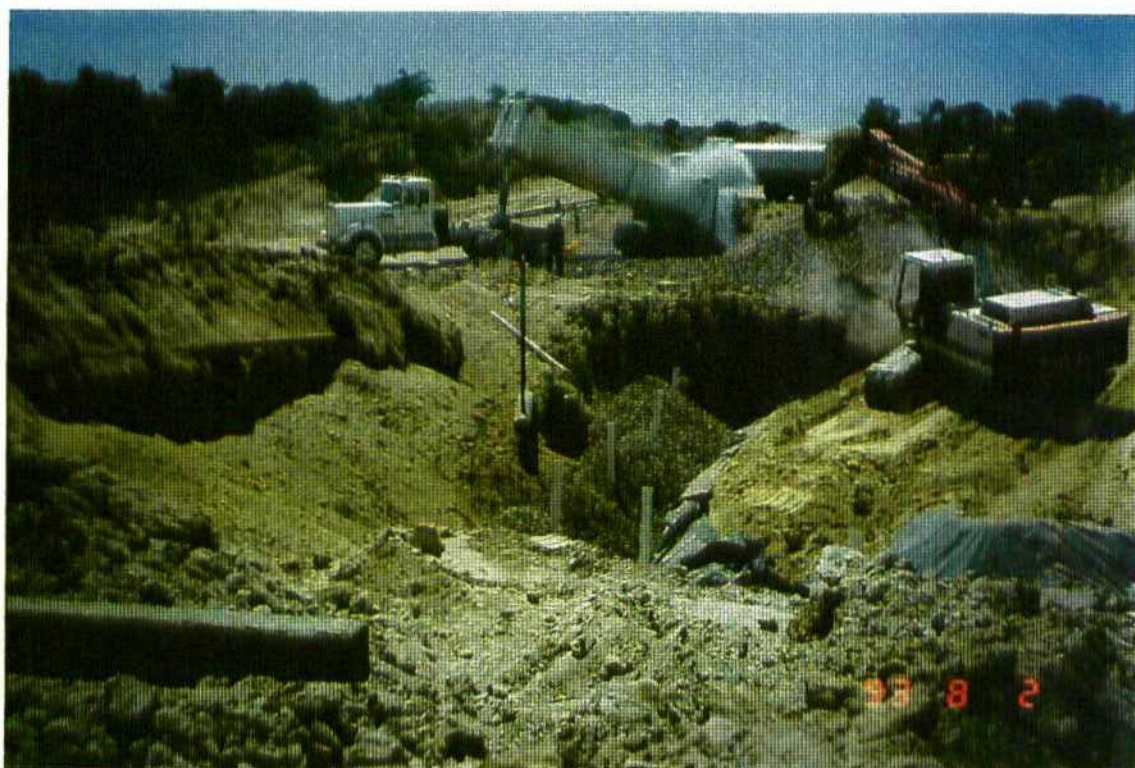
SOIL VAPOR EXTRACTION (SVE) SYSTEM INSTALLATION
