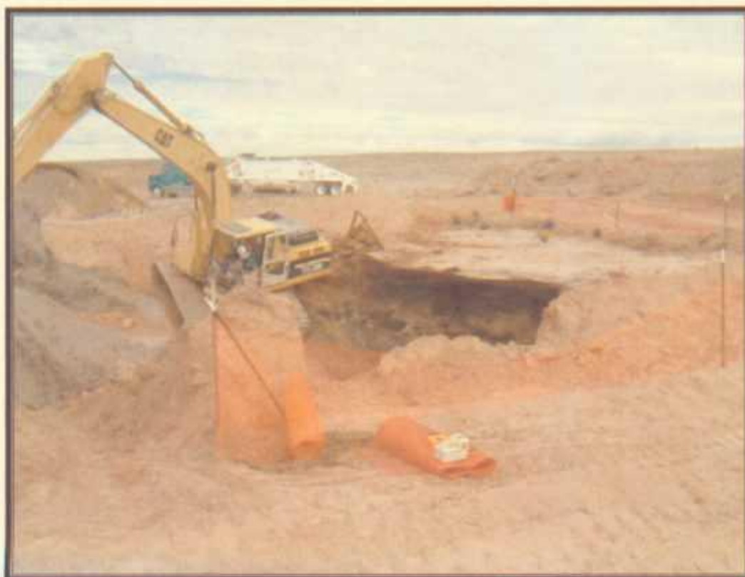
Photo 3: View to the north showing removal of hydrocarbon-impacted soil.
