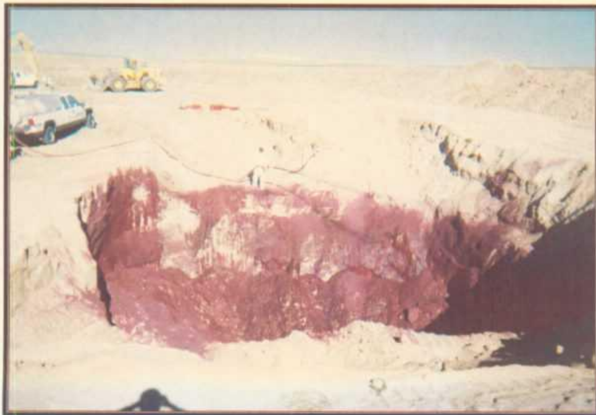
Photo 11: View to the north showing application of "oxidizer".
