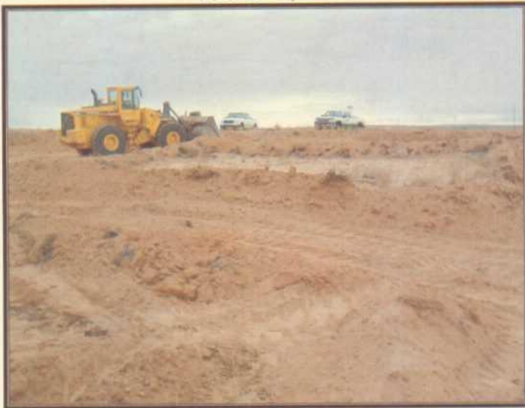
Photo 1: View to the south showing removal of the overburden
