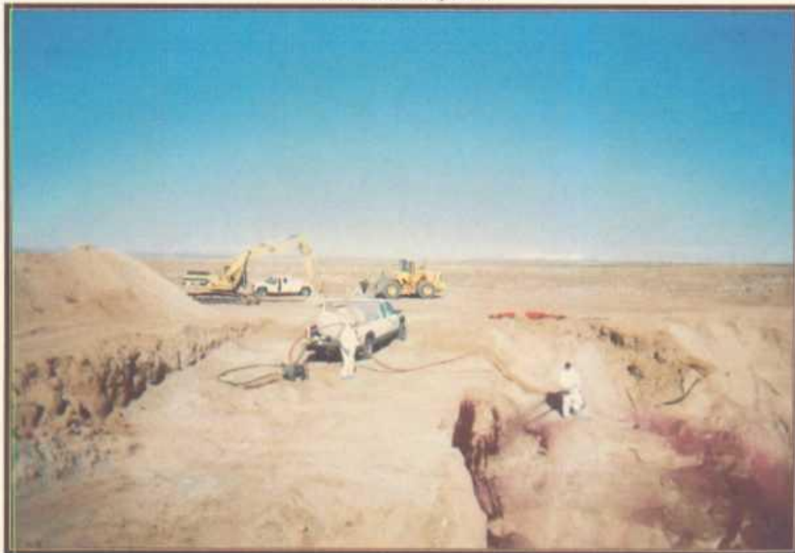
Photo 10: View to the north showing application of "oxidizer".
