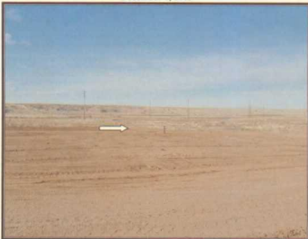
Photo 13: View to the west showing completion of backfill activities, final grade and MW-7.
