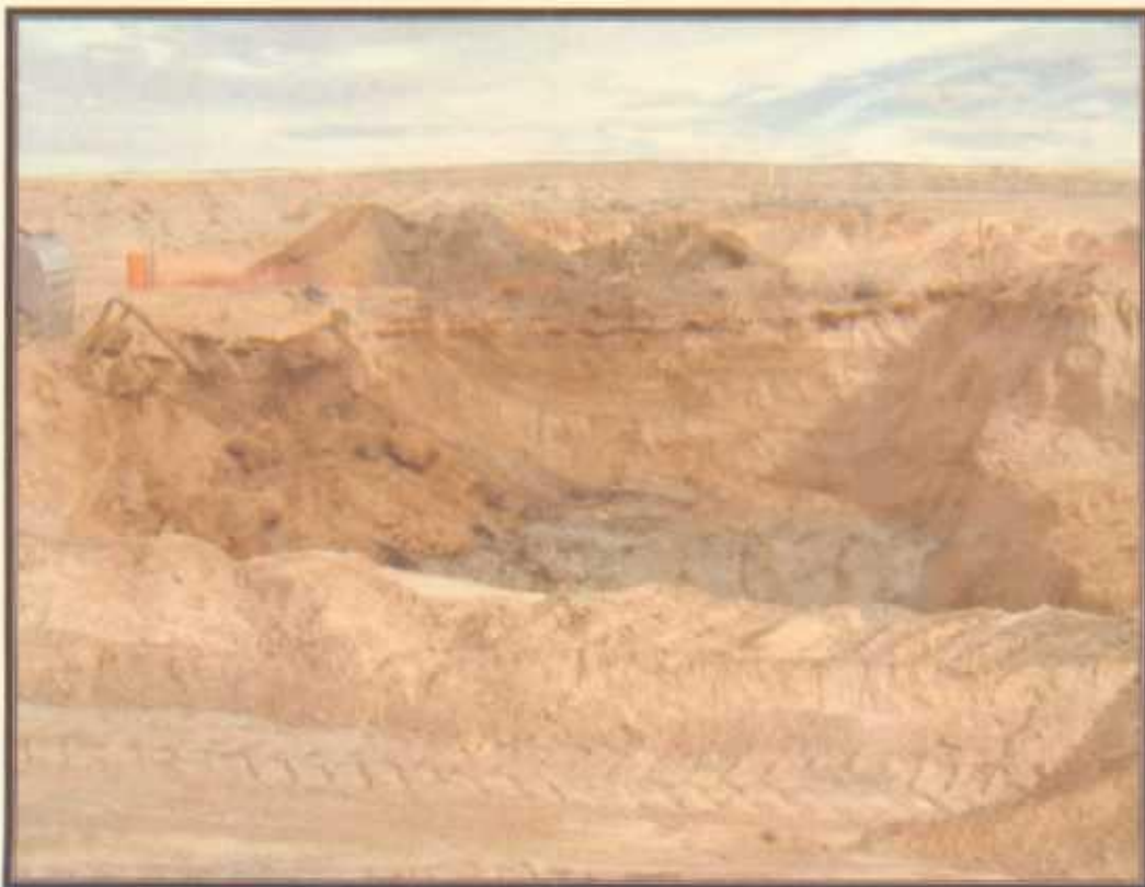
Photo 7: View to the east showing excavation area.
