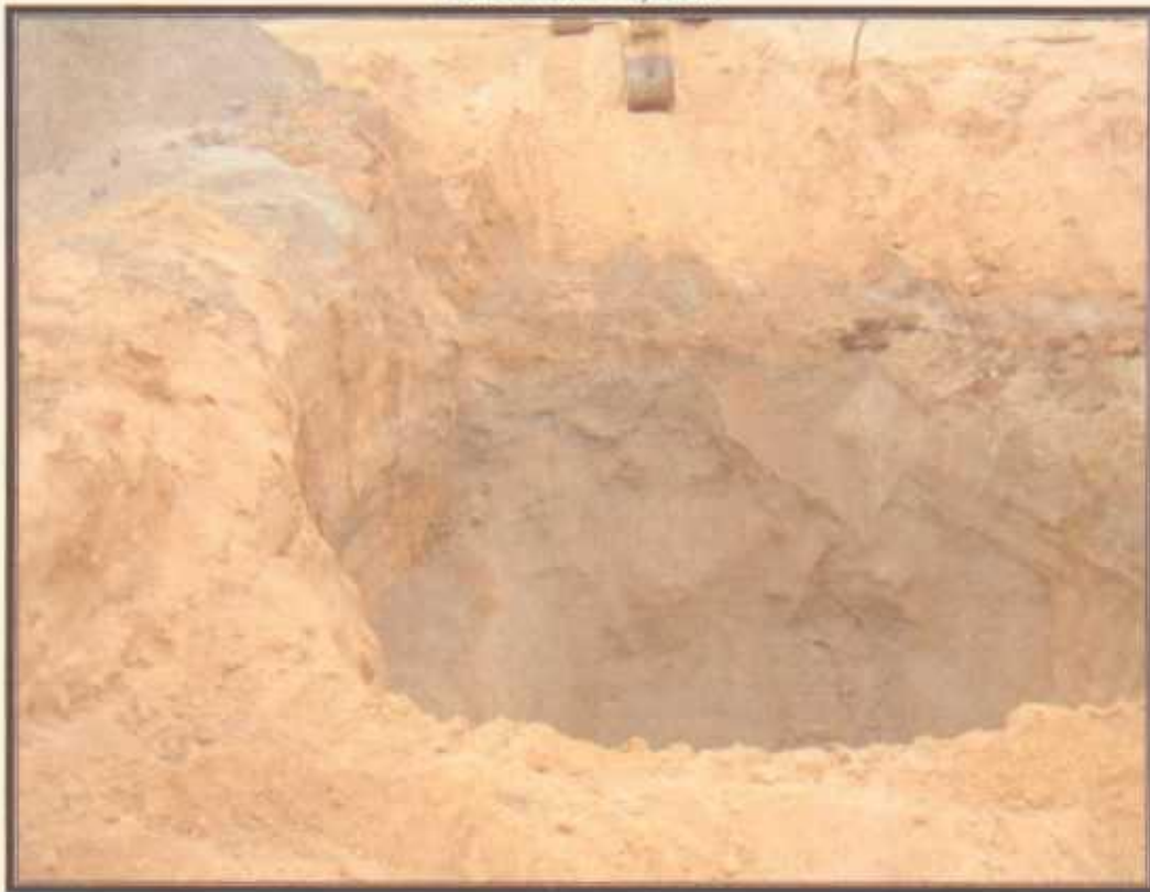
Photo 6: View to the north showing the excavation area.
