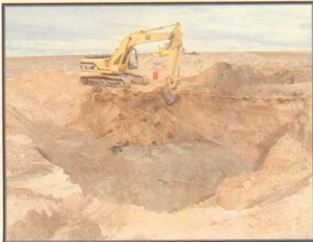
Photo 5: View to the northeast showing removal of the overburden.
