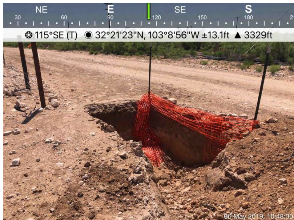
DP-19 Excavation Viewing Southeast, May 6, 2019
