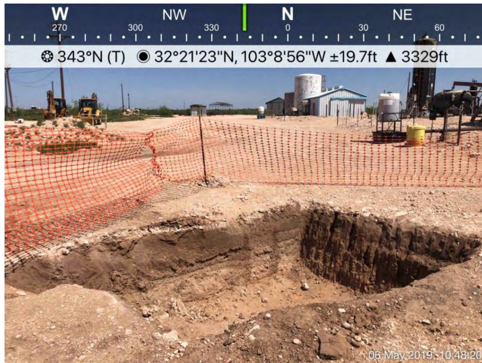
DP-20 Excavation viewing North, May 6, 2019
