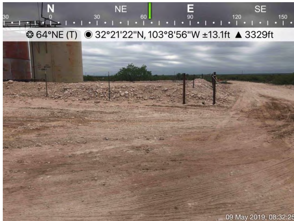
Backfilled Area near DP-19 viewing East, May 9, 2019
