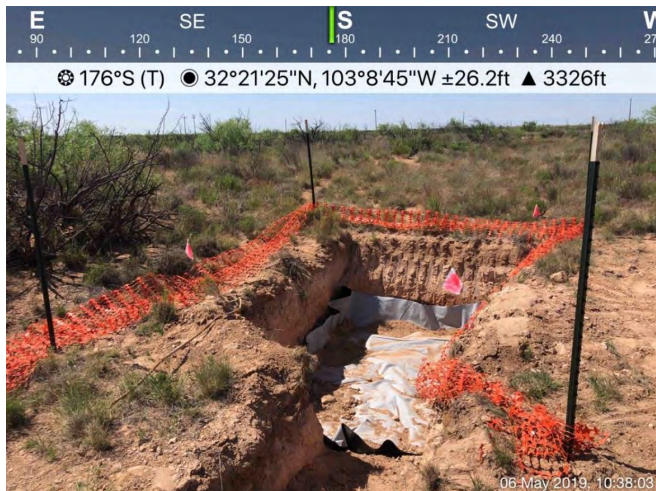
DP-12 Excavation Viewing Southwest, May 6, 2019
