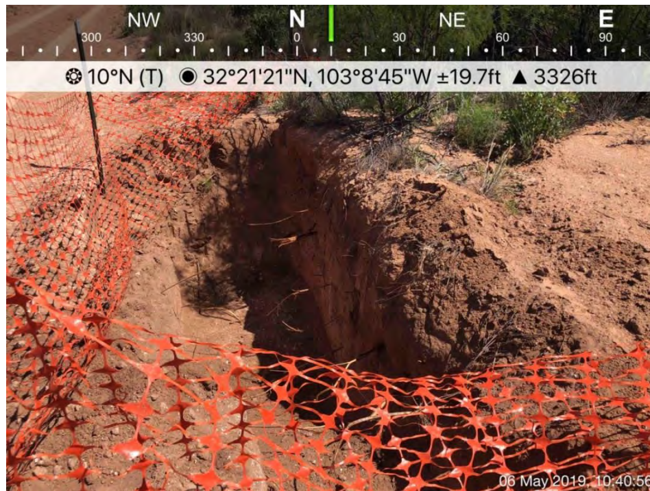
DP-4 Excavation Viewing North, May 6, 2019
