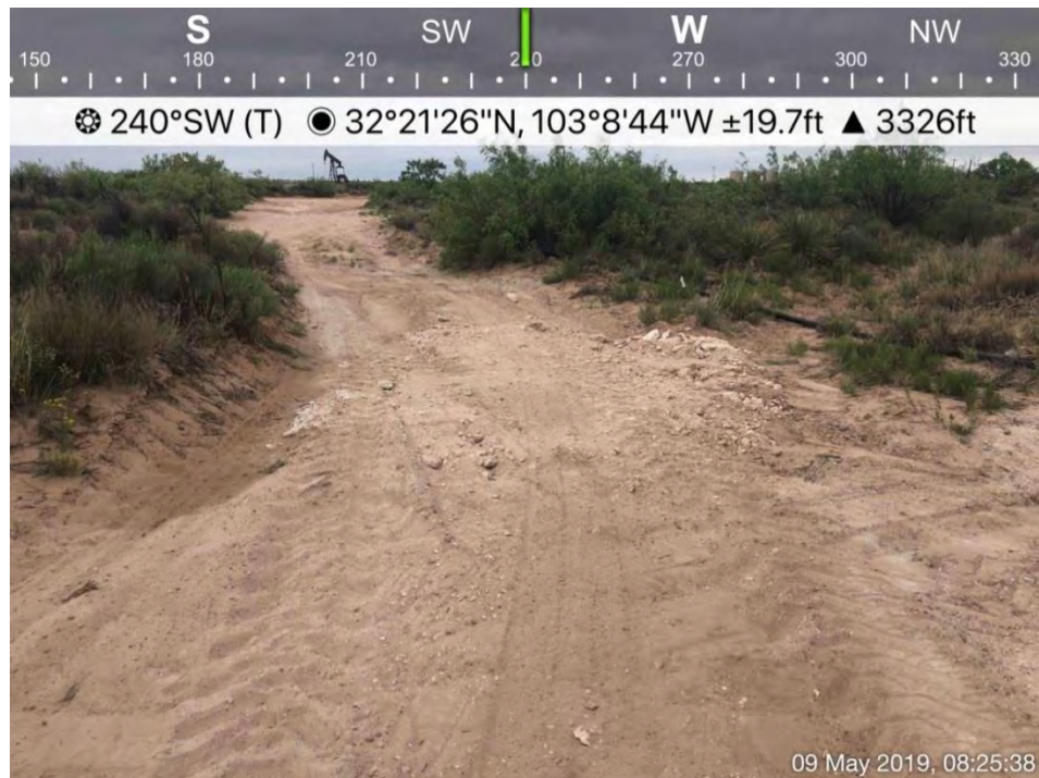
Backfilled Area near DP-11 Viewing West, May 9, 2019
