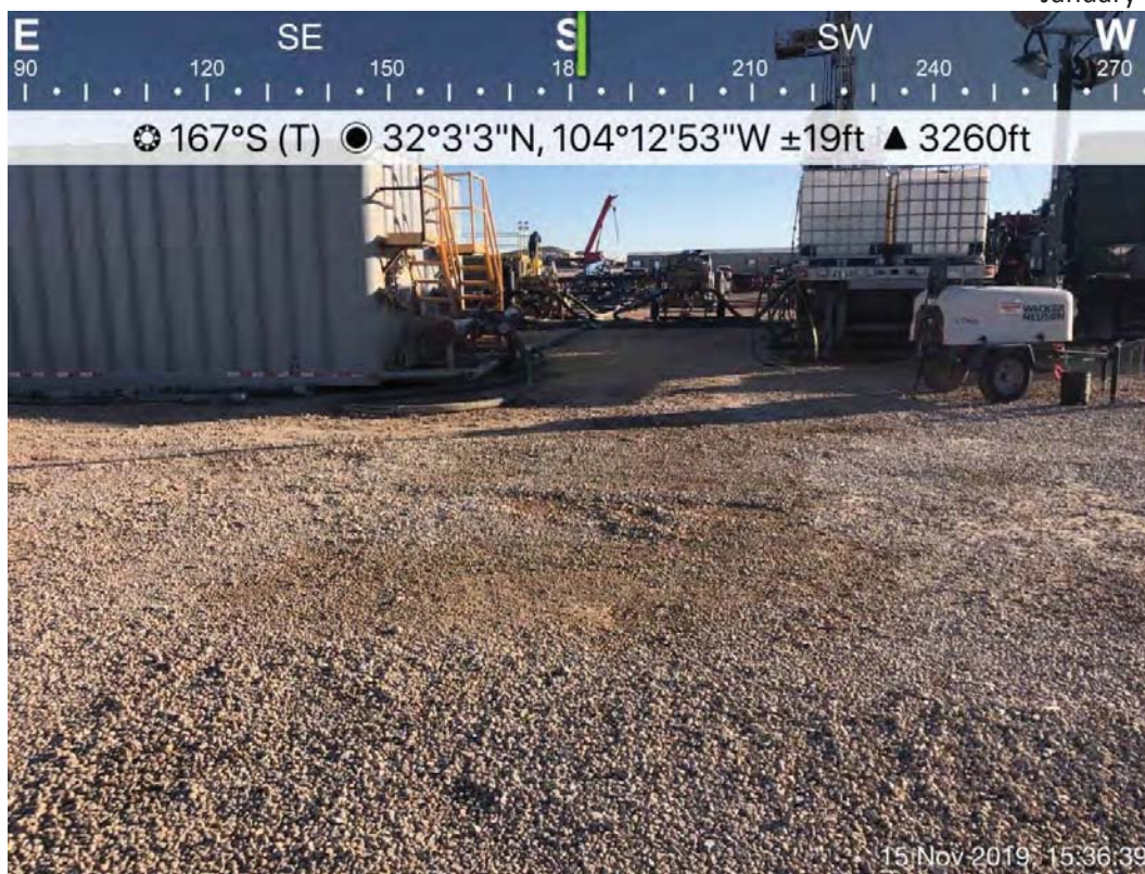
Diesel Spill Area Viewing South, November 15, 2019
