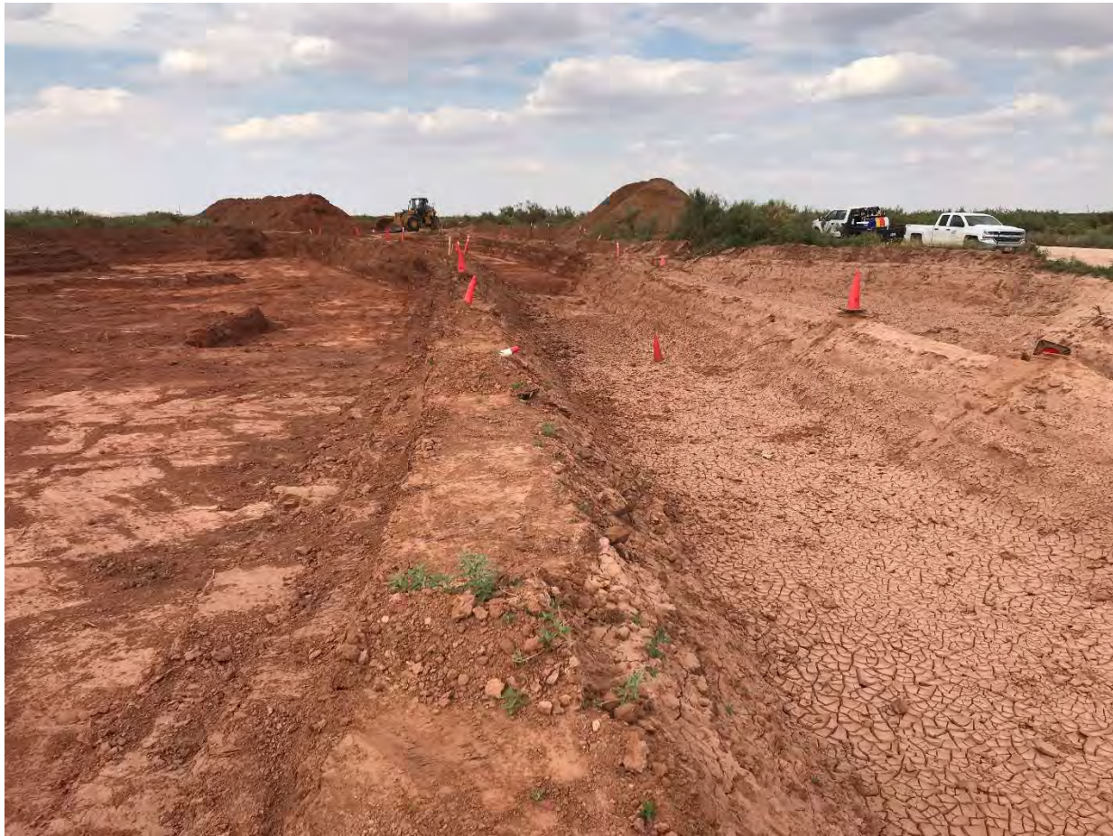
View of the final northern excavation area and deferred areas along the pipelines.
