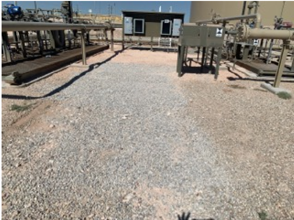
Backfilled Excavation – Facing North
