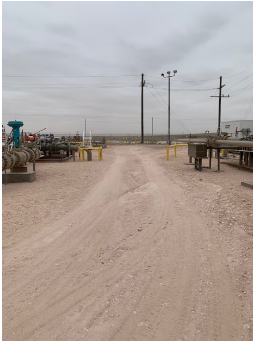
Backfilled Excavation – Facing South
