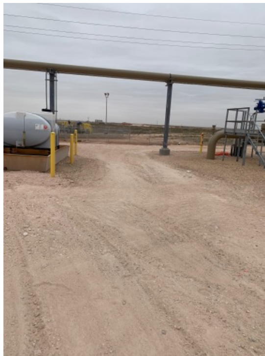
Backfilled Excavation – Facing West
