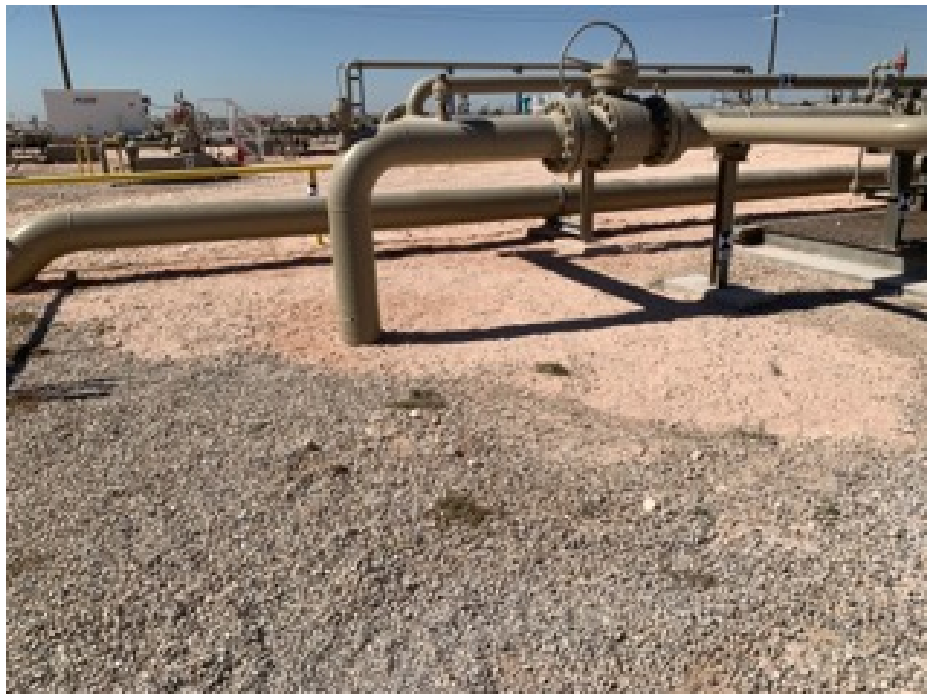
Backfilled Excavation – Facing West
