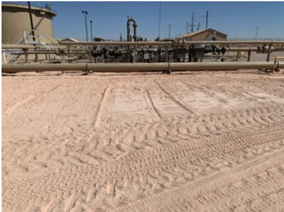
Backfilled Excavation – Facing East
