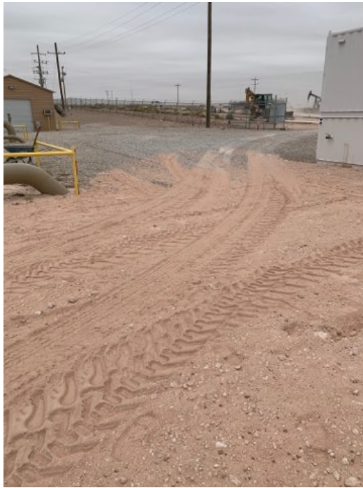
Backfilled Excavation – Facing Southeast
