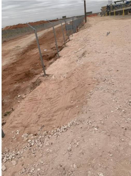
Backfilled Excavation – Facing North
