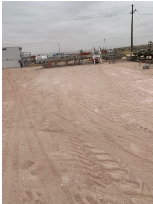
Backfilled Excavation – Facing South
