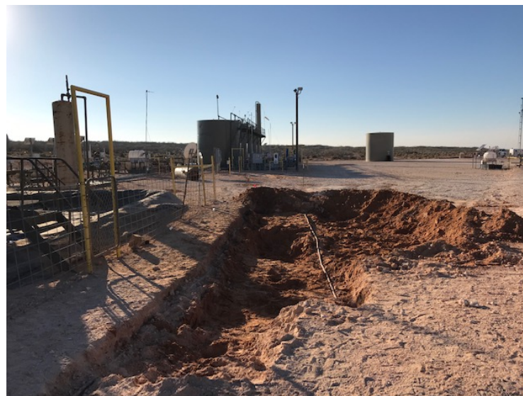
Photograph 2: West facing view of excavation north of process equipment.
