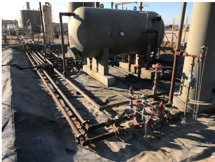
Photograph 1: Northwest facing view of lined process equipment containment.
