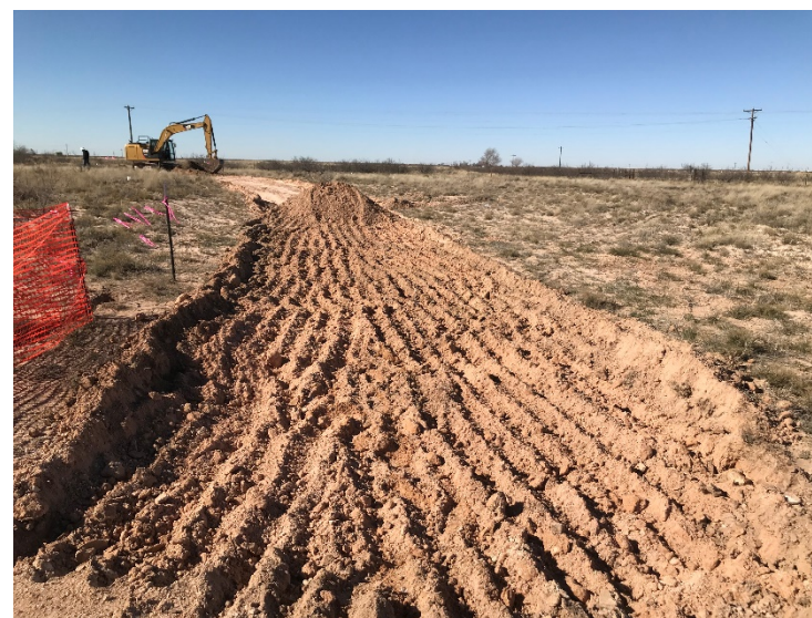
Photograph 4: View west of road excavation.
