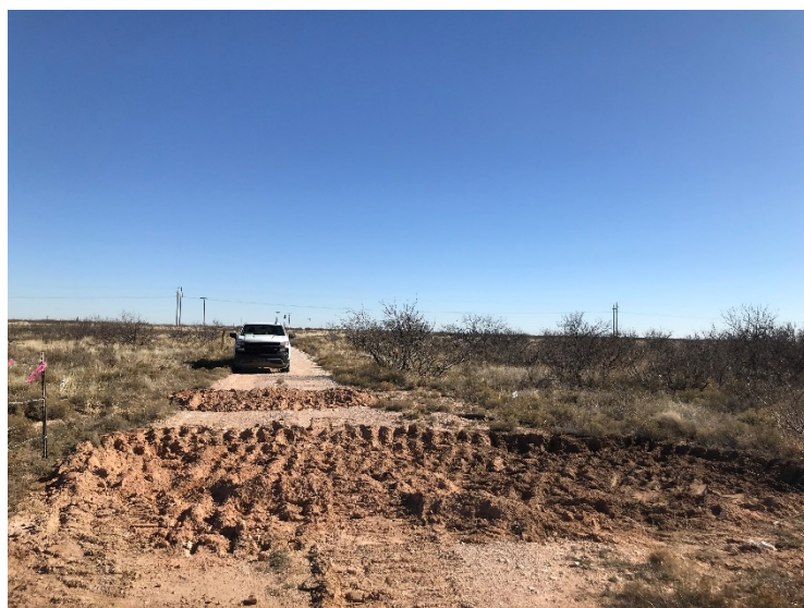
Photograph 3: View east of road excavation.
