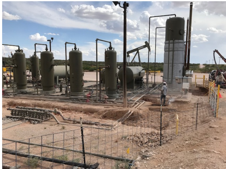
Photograph 3: South facing view of excavation.
