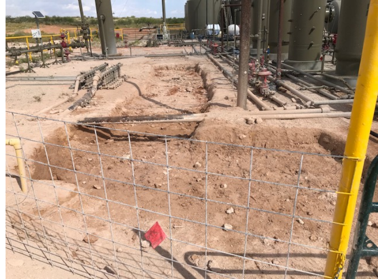
Photograph 2: East facing view of excavation.
