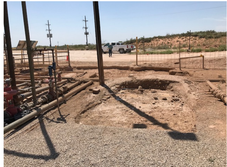
Photograph 4: West facing view of excavation.
