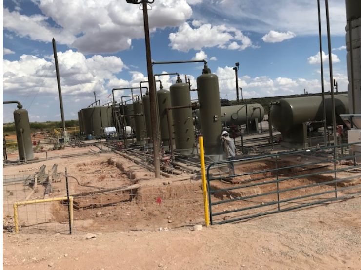
Photograph 1: East facing view of excavation.
