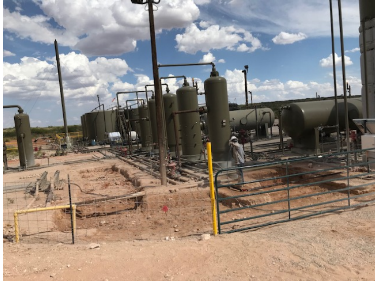
Photograph 1: East facing view of excavation.
