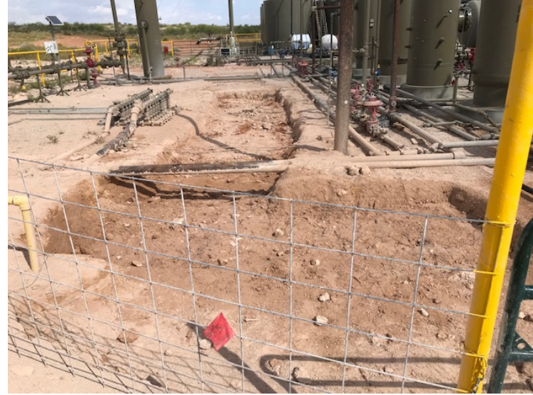
Photograph 2: East facing view of excavation.
