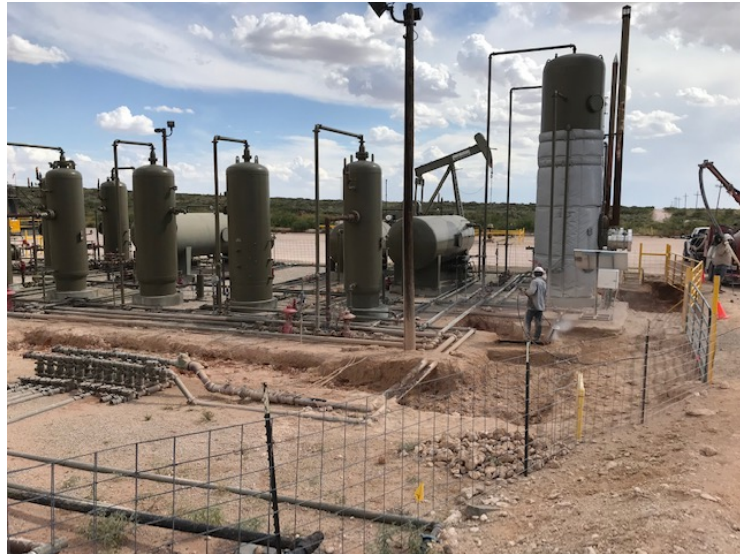
Photograph 3: South facing view of excavation.
