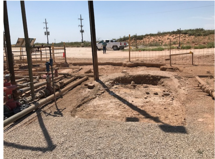
Photograph 4: West facing view of excavation.
