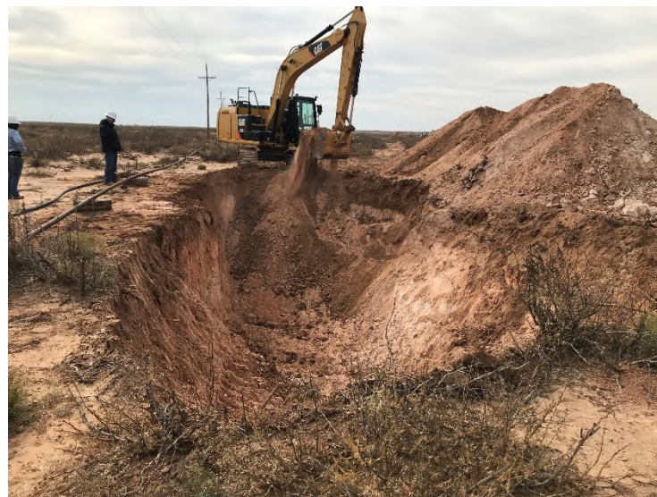
Photograph 2: Eastern view of site during excavation activities.
