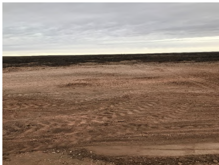
Photograph 4: View of backfilled excavation after re-seeding.
