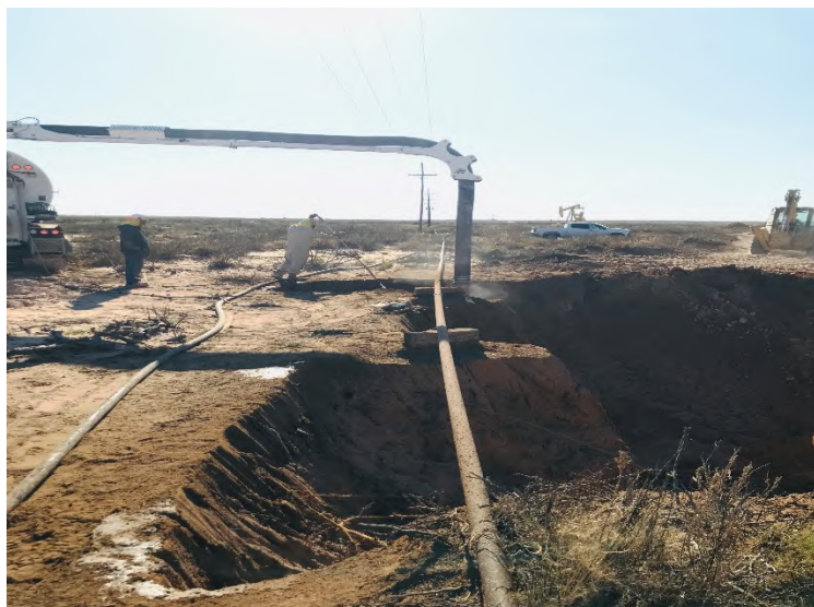
Photograph 3: Eastern view of site during Hydro-excavation activities.
