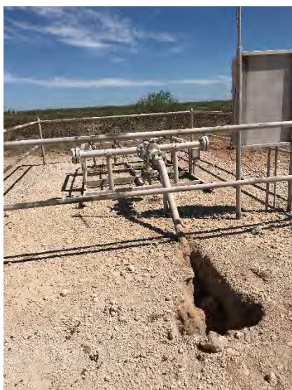
Photograph 3: View of hydrovac excavation around riser equipment facing north.
