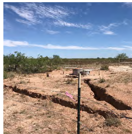
Photograph 4: View of hydrovac excavation around above ground equipment and active pipelines facing northeast.
