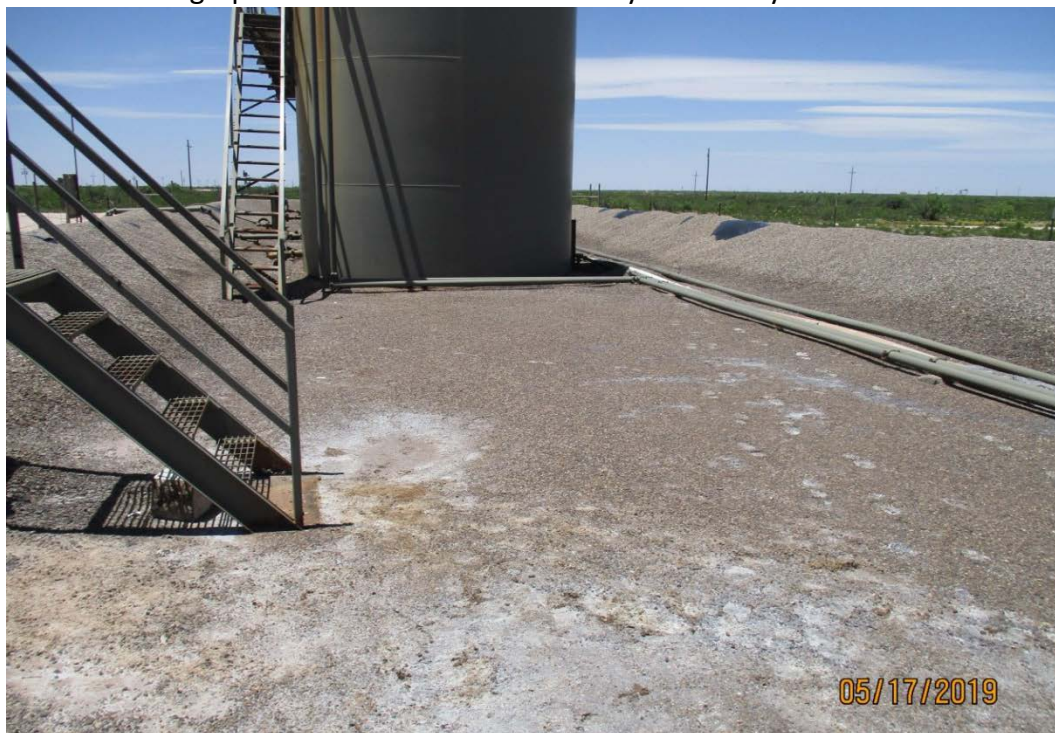
Photograph 1: Lea KG State Tank Battery Secondary Containment
