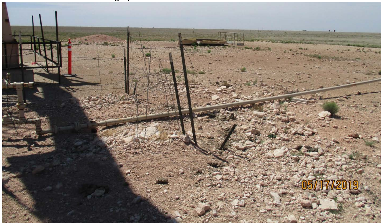
Photograph 4: Remediated Area North of Wellhead
