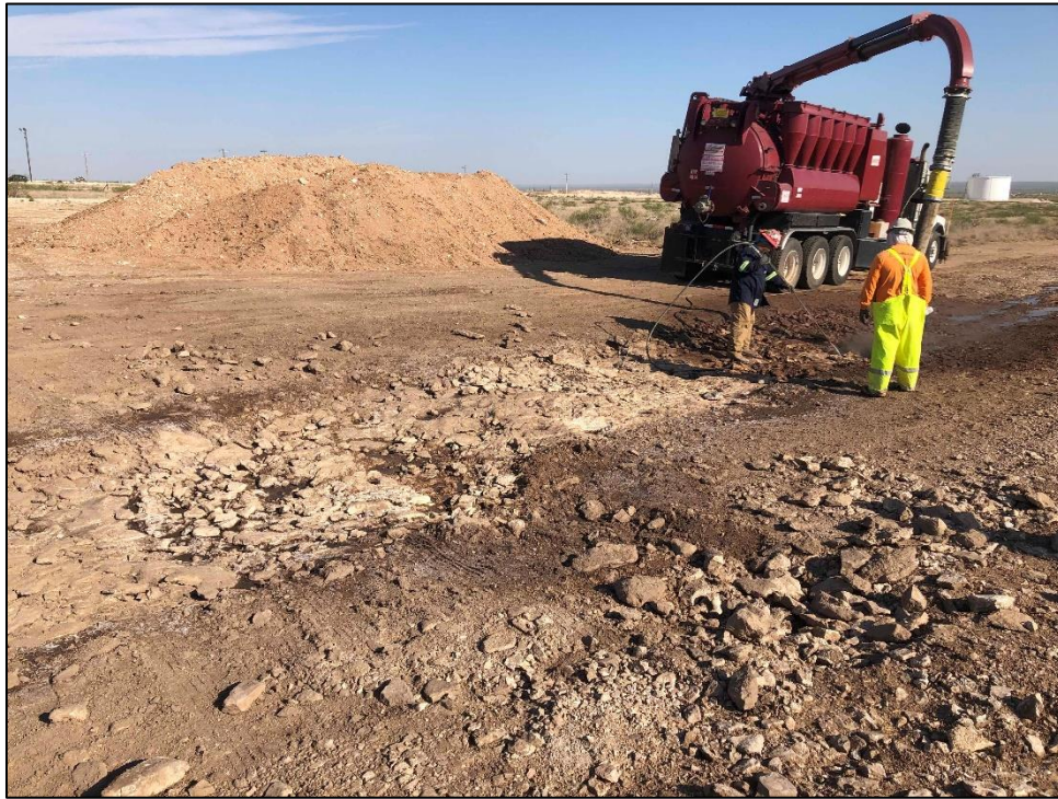
PHOTO 35: View of Hydro-excavation Activity, Facing West. 9/05/2019 / TIME: 10:40PM / GPS: 32.5261 -103.5206
