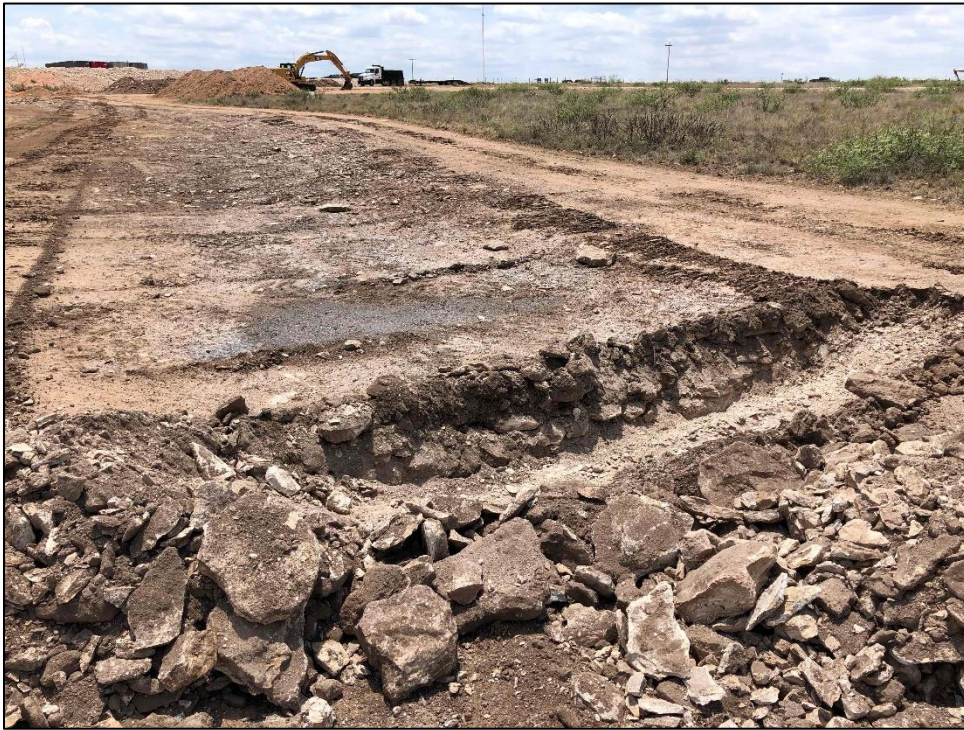
PHOTO 29: View of TT-2, Facing South. 7/23/2019 / TIME: 14:40PM / GPS: 32.5261 -103.5206
