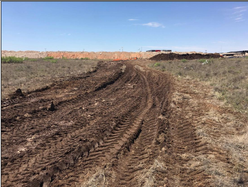
PHOTO 16: View of Remediation Activity, Facing South. 6/05/2019 / TIME: 12:20PM / GPS: 32.5261 -103.5206
