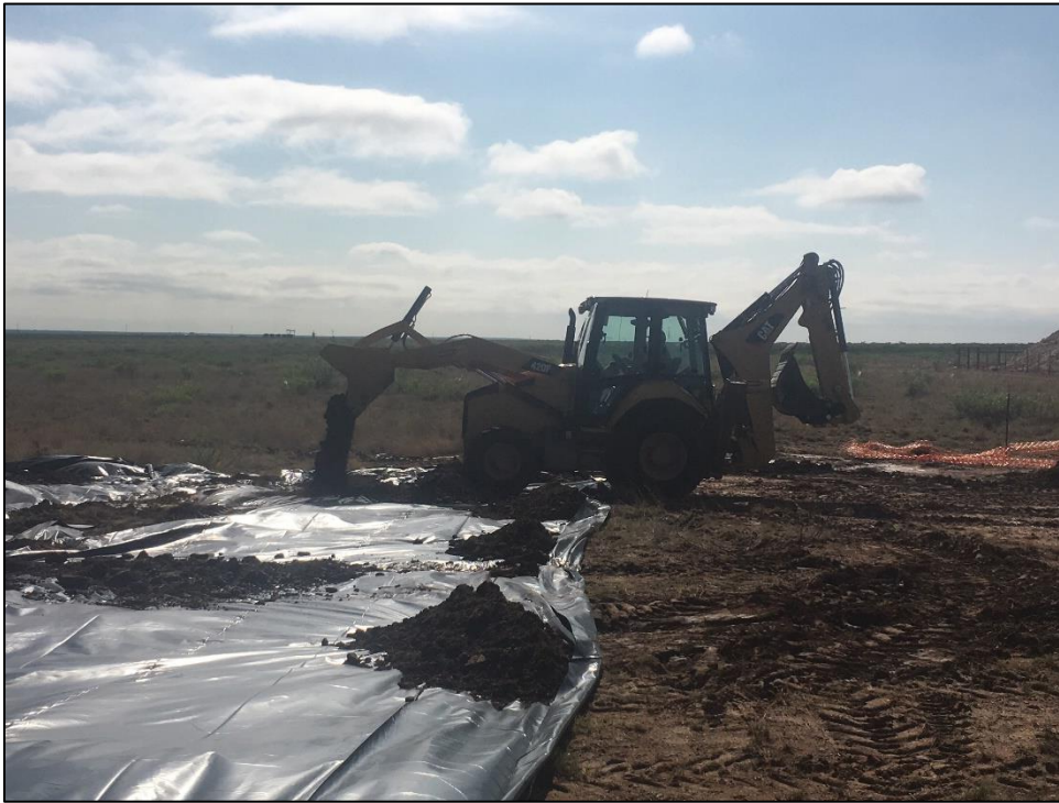
PHOTO 15: View of Remediation Activity, Facing East. 6/04/2019 / TIME: 10:04AM / GPS: 32.5255 -103.5211
