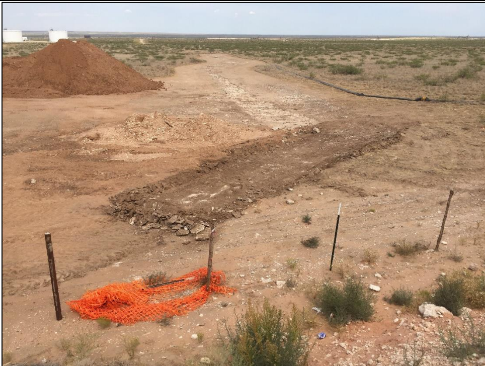
PHOTO 38: View of Completed Excavation, Facing North. 9/20/2019 / TIME: 13:19PM / GPS: 32.5261 -103.5206
