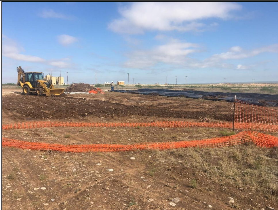
PHOTO 14: View of Remediation Activity, Facing West. 6/04/2019 / TIME: 10:01AM / GPS: 32.5253 -103.5207
