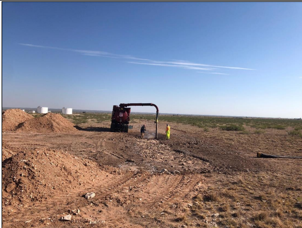
PHOTO 36: View of Hydro-excavation Activity, Facing North. 7/05/2019 / TIME: 10:30PM / GPS: 32.5261 -103.5206
