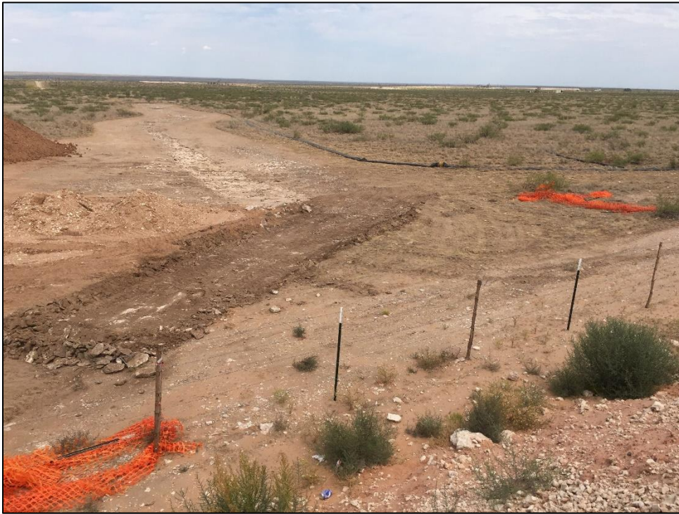
PHOTO 37: View of Completed Excavation, Facing Northeast. 9/20/2019 / TIME: 13:20PM / GPS: 32.5261 -103.5206
