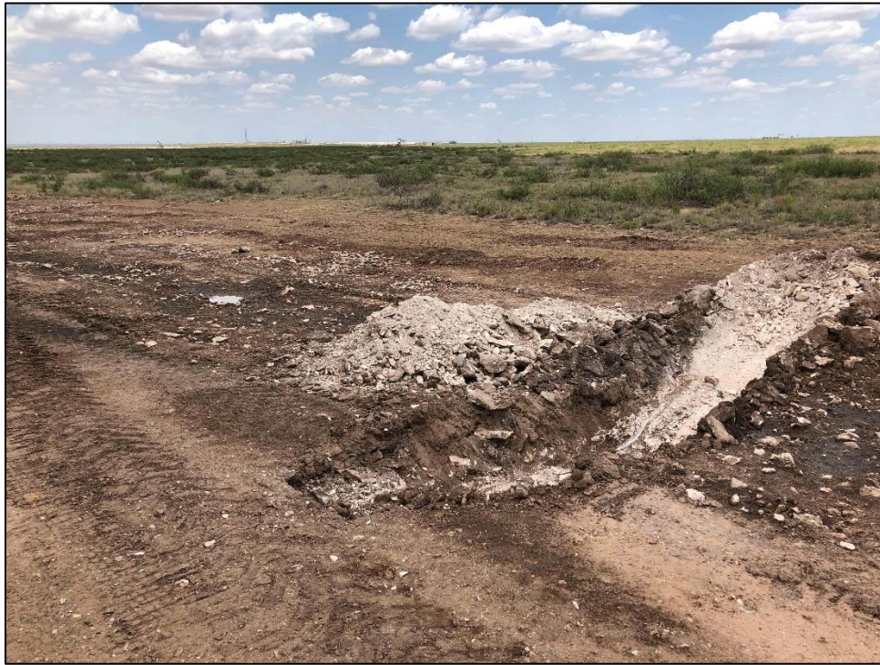
PHOTO 31: View of TT-1, Facing Northeast. 7/23/2019 / TIME: 13:51PM / GPS: 32.5261 -103.5206
