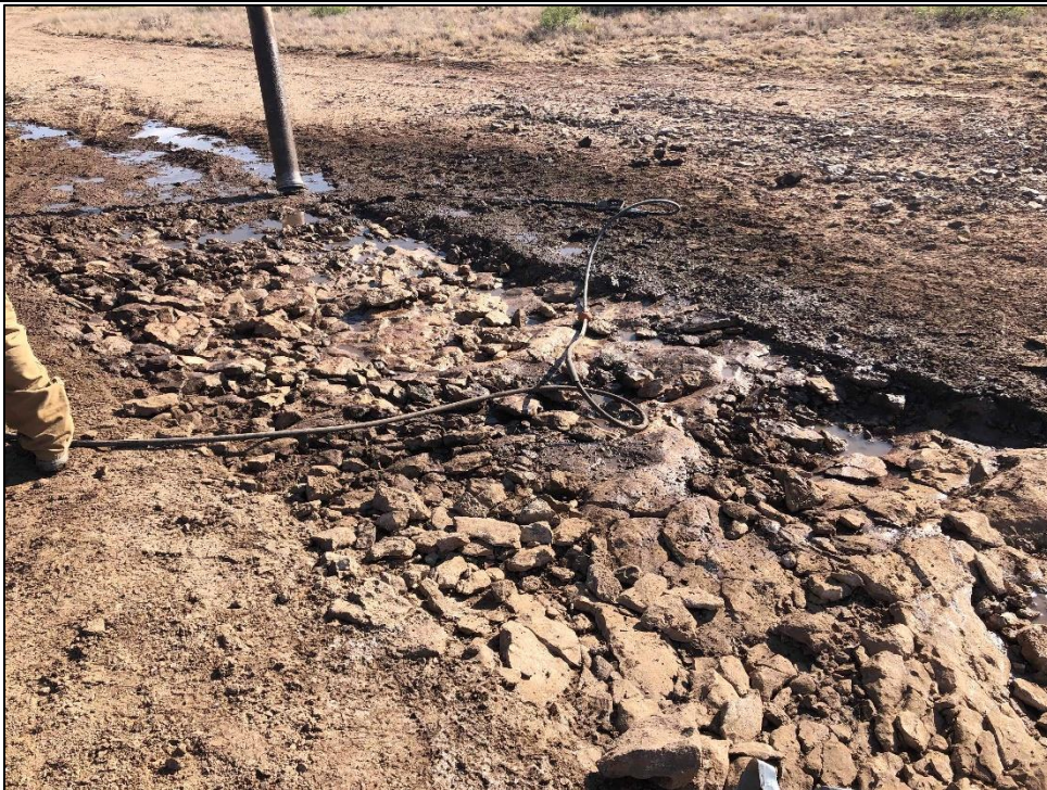
PHOTO 34: View of Hydro-excavation Activity, Facing North. 9/05/2019 / TIME: 10:20PM / GPS: 32.5261 -103.5206
