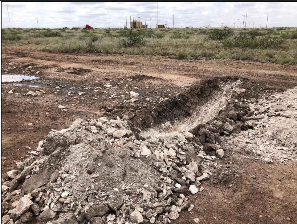
PHOTO 30: View of TT-3, Facing West. 7/23/2019 / TIME: 13:51PM / GPS: 32.5261 -103.5206
