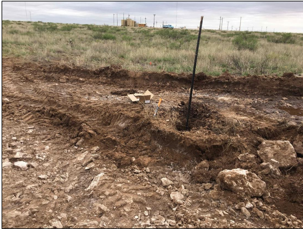
PHOTO 21: View of CS-8, Facing West. 6/10/2019 / TIME: 1:21PM / GPS: 32.5272 -103.5202
