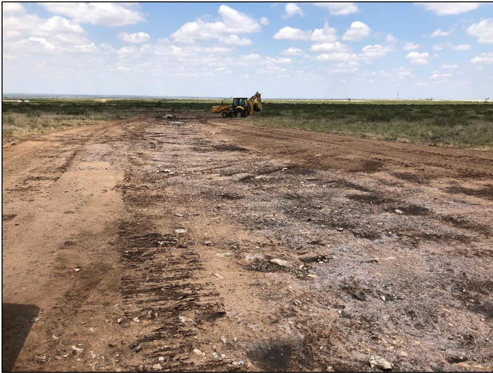
PHOTO 33: View of backfilling trenches, Facing North. 7/23/2019 / TIME: 14:42PM / GPS: 32.5261 -103.5206
