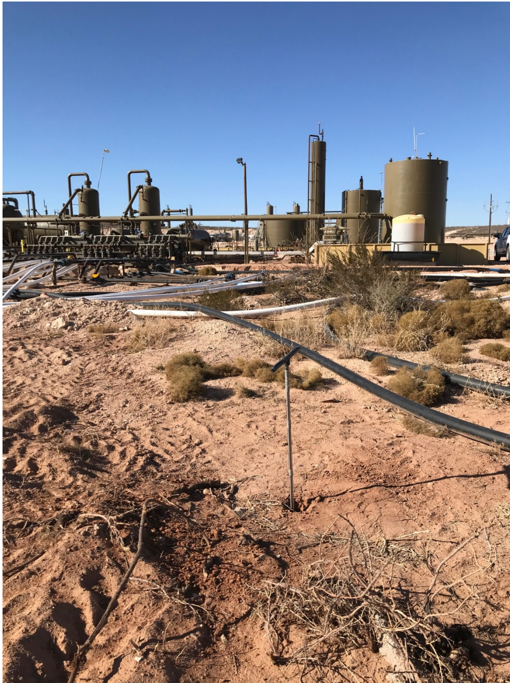
Photograph 5: North facing view of overspray area south of the pad, during assessment activities.
