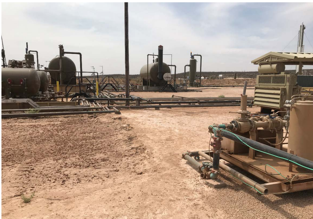
Photograph 4: View of excavation area.
