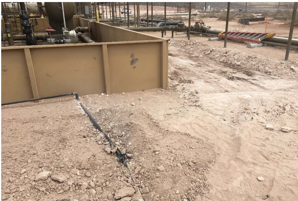
Photograph 2: View of excavation area.
