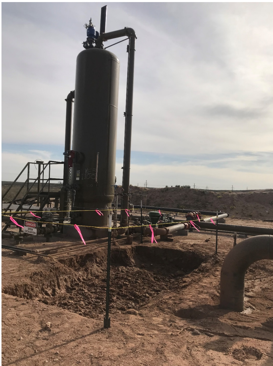
Photograph 5: View of excavation area.
