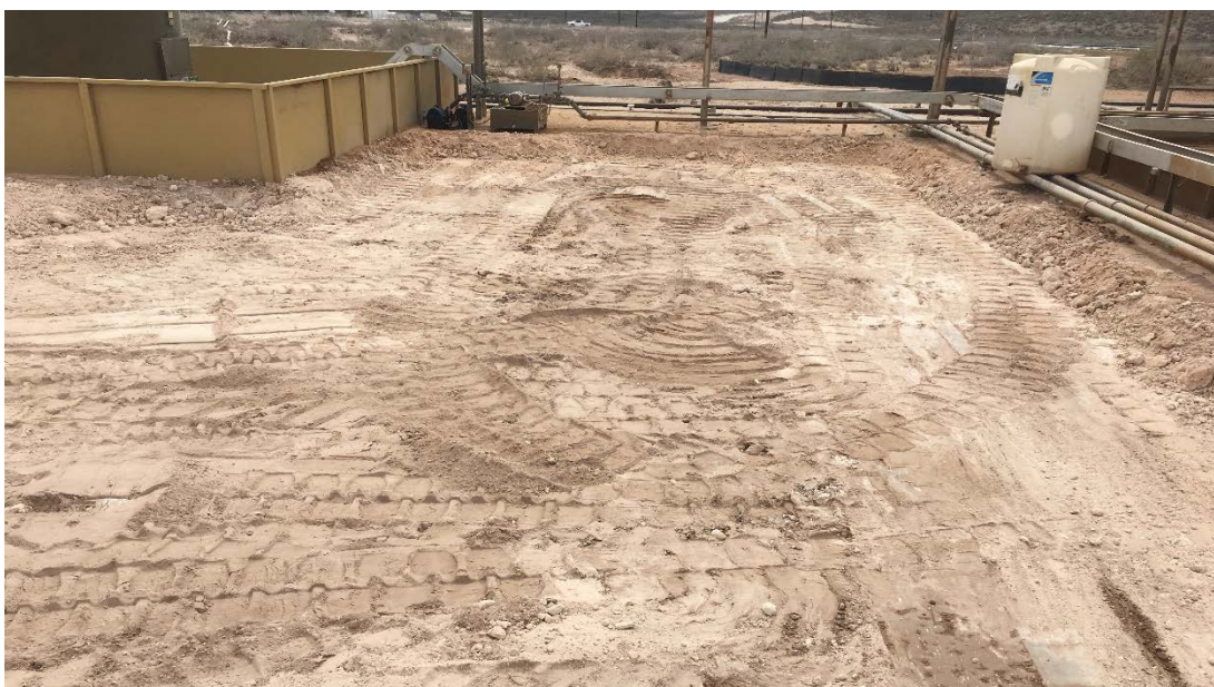
Photograph 3: View of excavation area.
